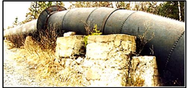
View of another expansion joint and bend near powerhouse.
