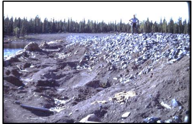
View of failed side dam.
