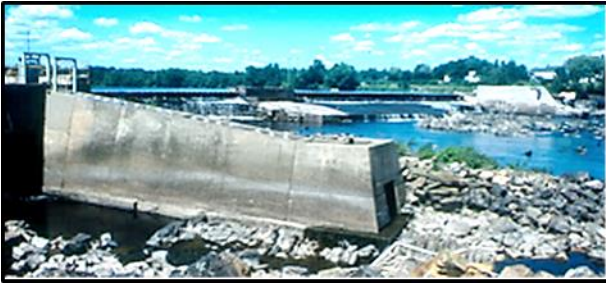
View of stoplog-controlled weir at the hydro plant.
