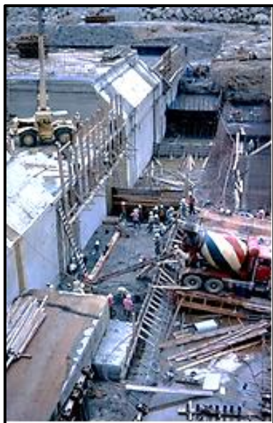
View of downstream toe of concrete dam showing 45 degree slope.
