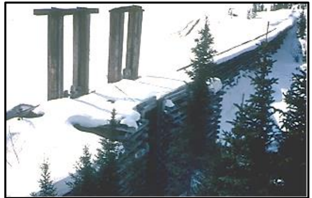
Timber sluice gates and part of timber crib dam.
