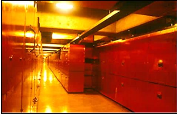
The “gold” room – copper-enclosed switchgear
