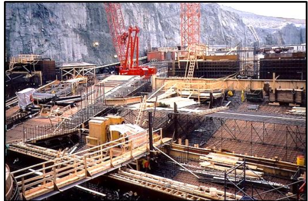
Draft tube formwork and reinforcing.
