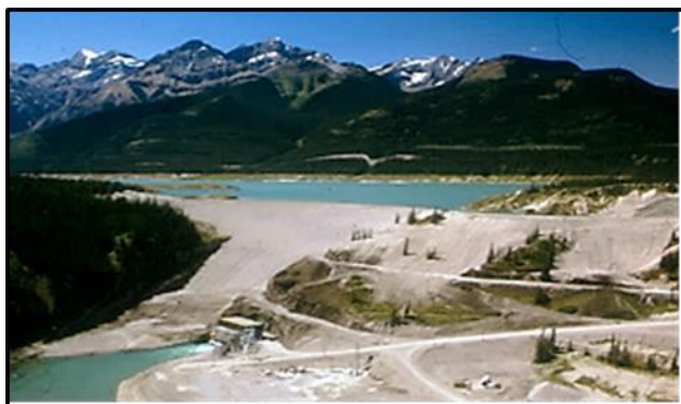
Aerial view of dam and powerhouse. Note large toe berm on dam to counter seepage.
