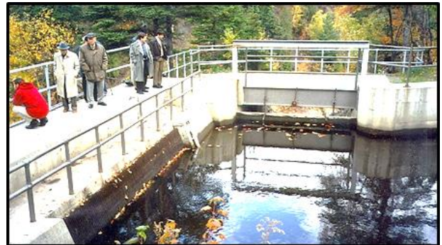
Hydro-Fraser spillway and canal intake structure.
