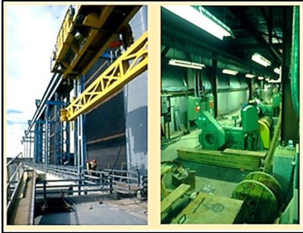
Left – spillway hoist structure. Right – interior of hoist house, hoists still being installed.
