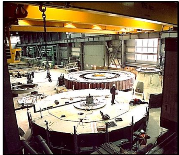
Assembling generator rotors. Below - powerhouse generator floor.
