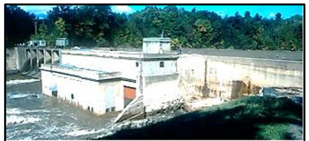
Powerhouse flooded from debris in river bed.
