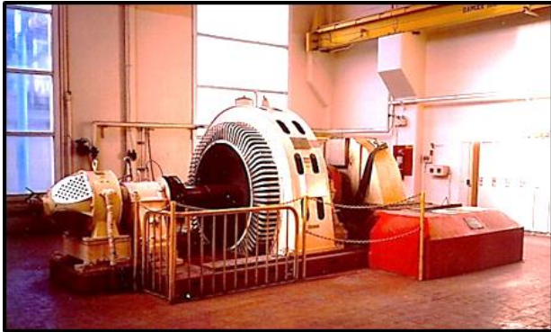
Horizontal axis 2-jet impulse unit, installed in 1947.
