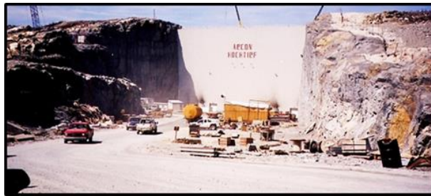
Giant hoarding for winter intake construction.
