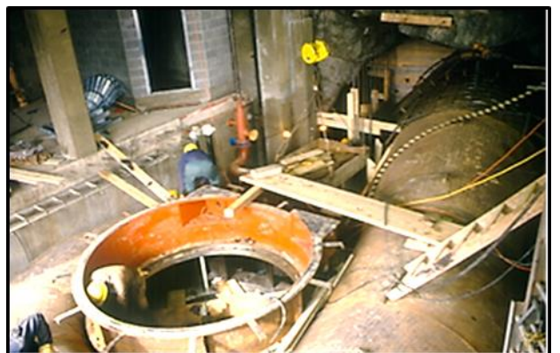
Spiral casing for turbine. Tunnel access door top left.
