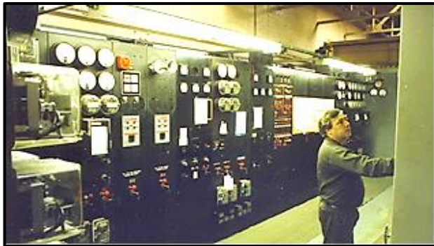
Ancient slate panel mounted instruments in control room.
