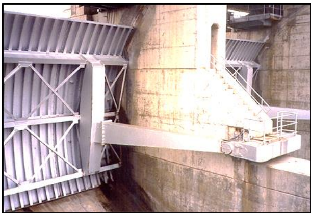
Tainter gate and arm to bearing support.
