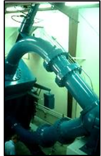
Impulse turbine at first powerhouse.
