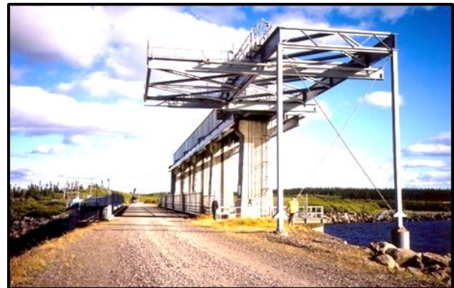
Below - View from left abutment. Note stoplog hoist monorail, but no monorail hoist.
