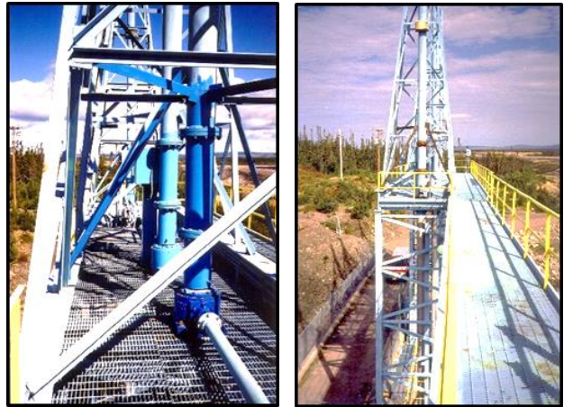
Two views of screw stem hoists on spillway gates.
