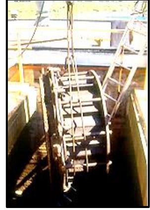
Left- powerhouse interior. Right - Turbine distributor being removed for repairs.
