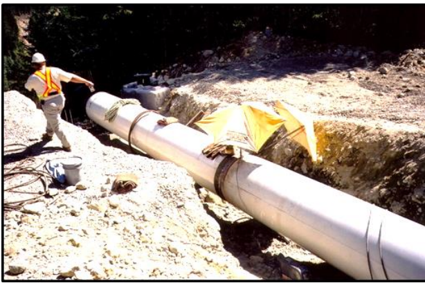
Pipe aligned and ready for welding.
