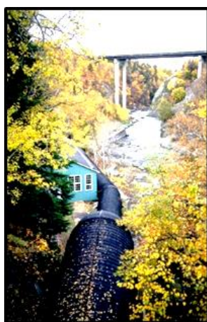
Wood stave pipe to Hydro-Fraser powerhouse.
