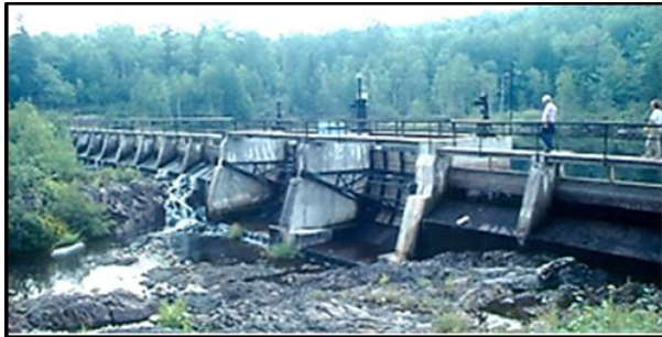
Tainter gate and stoplogs at Nictaux. Note hand crank hoists at each pier and timber strut a center of stoplogs to prevent lifting.
