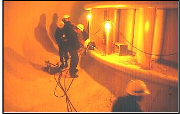
Junction of 6.25m penstock to turbine spiral casing.
