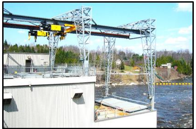
Cranes retrofitted to powerhouse.
