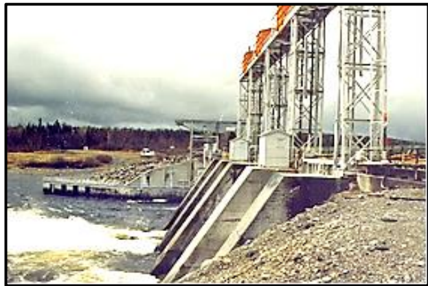
View of main spillway. Fish pass in middle left.
