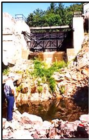
Cleared downstream slope at Lumsden Dam.
