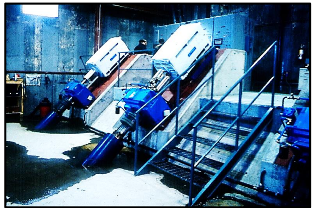
Inclined shaft generators and gearboxes.
