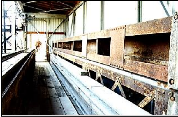
Stoplogs for spillway gates.
