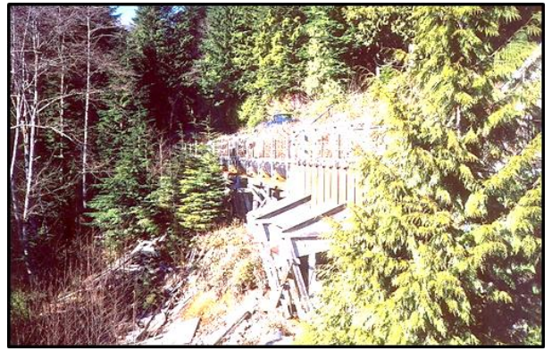
Flume, with bottom gravel sluice.
