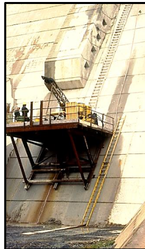
Slot cutter on left, finished slot on right.
