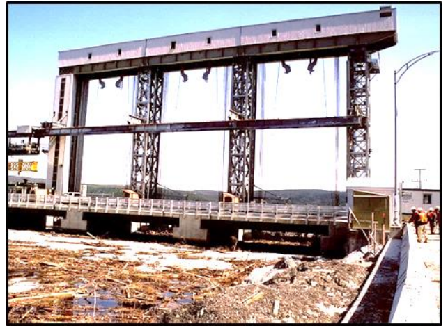
Spillway hoist structure. Full headpond. Note debris.
