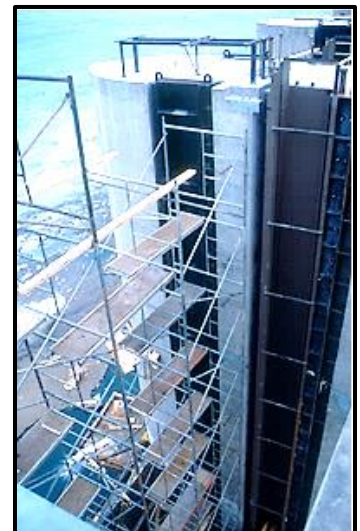
Downstream face – note new spillway piers.
