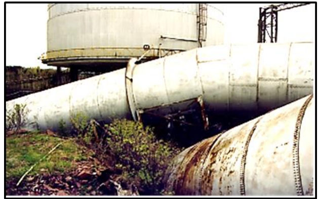
Penstock cross-over at surge tanks. Note bellows expansion joint.
