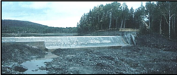
New spill weir downstream of dam breach.
