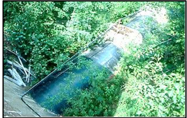
Riveted steel penstock at intake.
