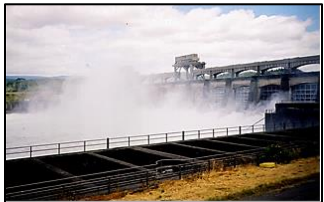
Spillway open to pass fish. Fish ladder in foreground.
