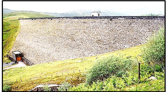
The Quoich concrete faced rock fill dam.
