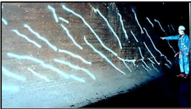
Me, pointing to painted crack pattern on casing wall.
