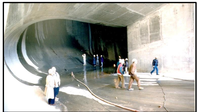
Looking into half of draft tube. Note enormous size!
