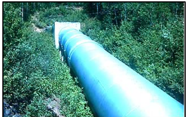
Welded steel penstock.
