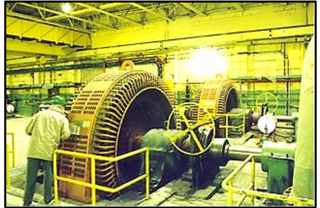
Double runner Francis units in second powerhouse.
