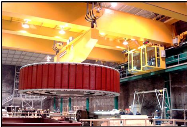
Two cranes installing generator rotor. Source – Hydro Quebec.
