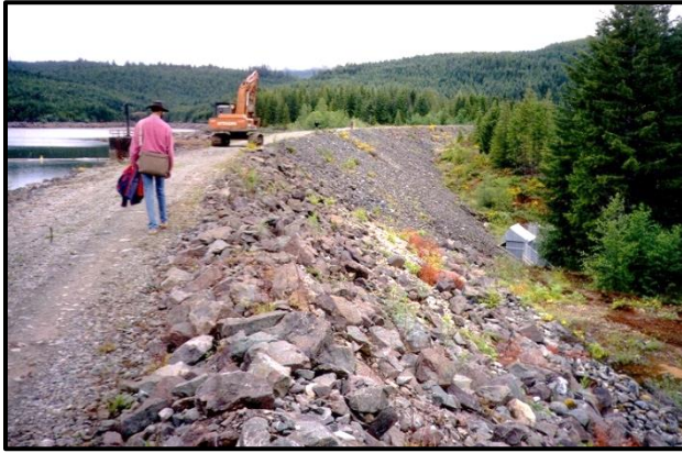
Embankment dam – slope to be flattened. Tower on left of Ray Stewart, outlet on right.
