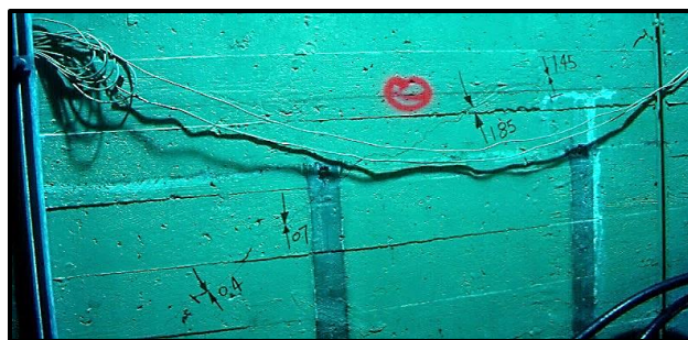
Monitoring 45 degree cracks inside powerhouse.
