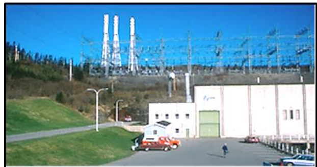
6-unit Bay d’Espoir powerhouse and surge tanks.
