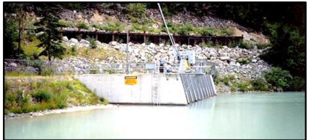
Intake with trash rake.
