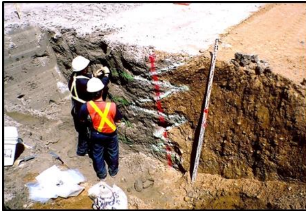
View of excellent “pine-tree” contact filter to core.
