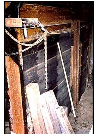
Old intake gate and air vent.
