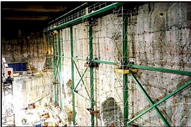
Powerhouse gallery upstream wall – note steel columns and man in center platform directing crane.
