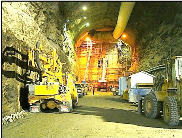
Diversion tunnel plug.
