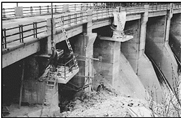
View of concrete platforms on every second pier.
