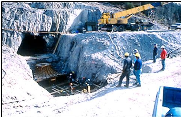
Powerhouse foundation – steel elbow for draft tube.
