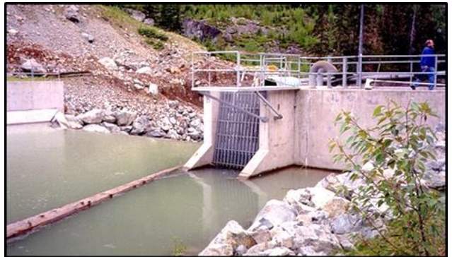
Automatic low level sluice – opens when units are closed.
