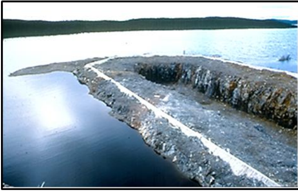
Completed bathtub spillway.
