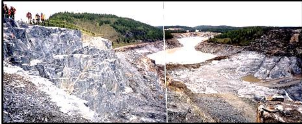
Abutment notch excavation, drained lake. Dyke LE-24A.
