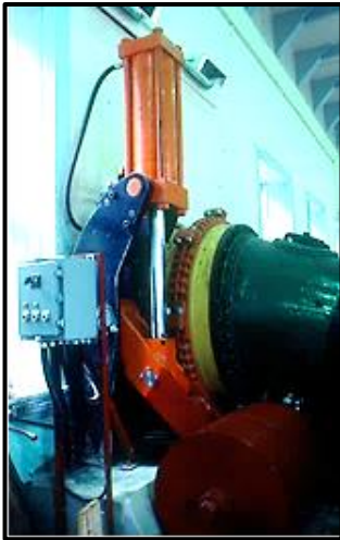
Inlet valve with servomotor on top,
