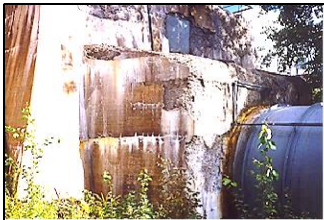
View of deteriorated concrete at penstock junction.
