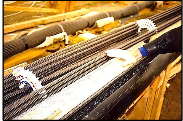
Assembling anchors.
