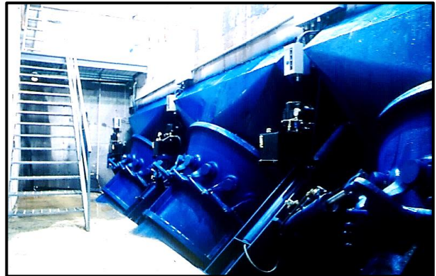
Inclined axis turbine units.
