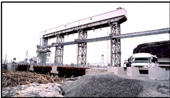
Completed spillway hoist structure. Note driftwood upstream of gates.
