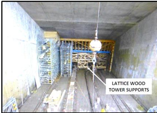
Photo showing lattice timber supports
