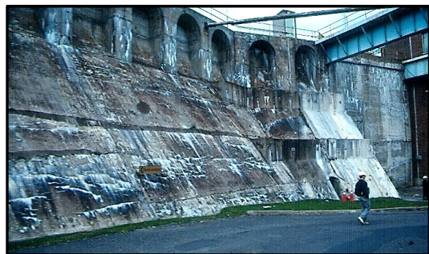
Old 1932 east abutment wall with AAR.
