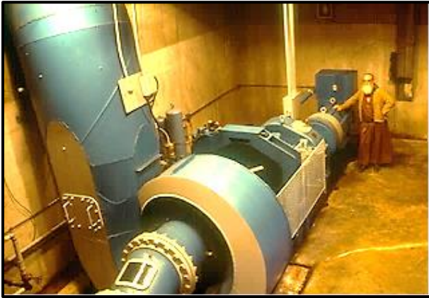
Kaplan turbine and 300kW generator.
