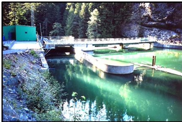
Mamquam weir and low level Tainter sluice gate.
