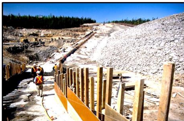
Forms for the concrete toe plinth.
