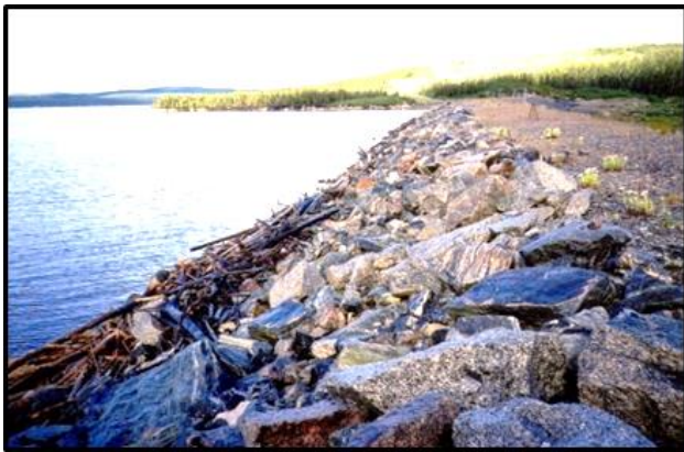
Rip-rap at side dam just west of bathtub spillway.
