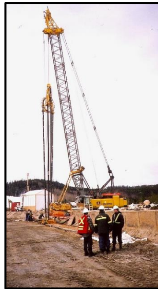
Bauer rig on panel excavation at Dyke A.
