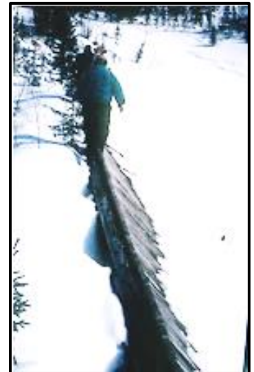
Timber sluice gates and part of timber crib dam.
