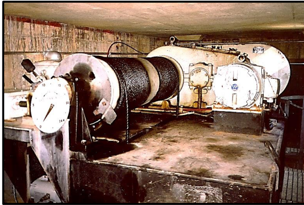
Intake gate hoist on steel beams just below deck.
