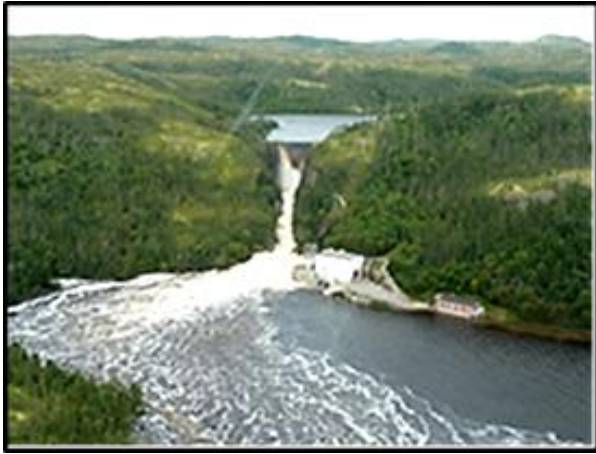
View of project just after the Igor hurricane had passed over – caused 1/5,000 flood. Sept. 2010. Note powerhouse level.
