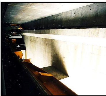
Draft tube hoist gallery – hoist capacity = 25 tons.
