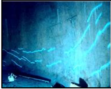
Cracks sloping down to middle in casing.
