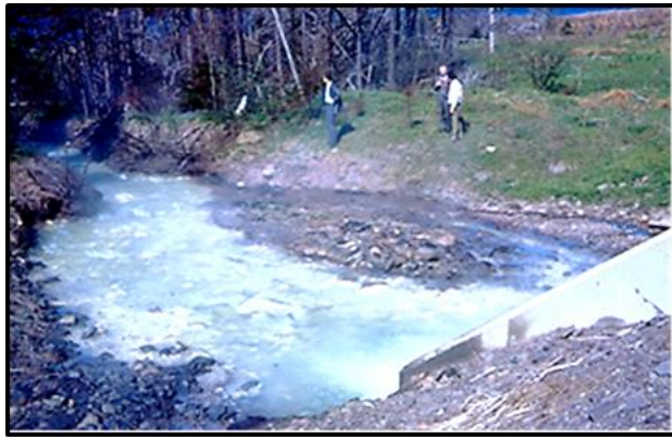
Excessive erosion at process water outlet.
