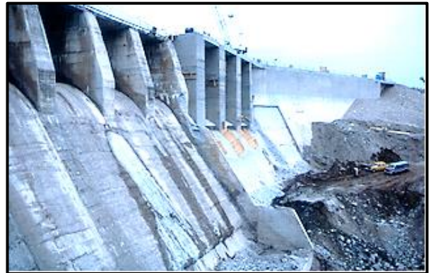
Downstream face – note new spillway piers.
