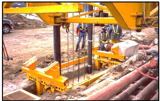
Interlocking panel excavation at Dyke A.
