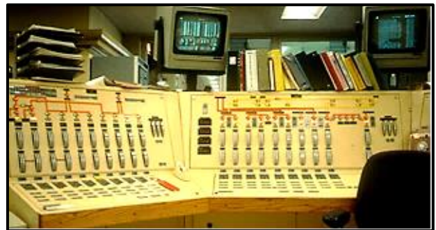
Powerhouse #2, analogue control room panel.
