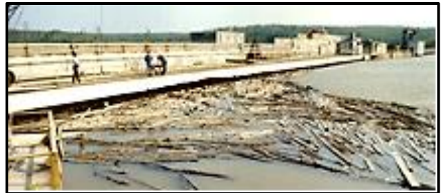
View of forebay. Top of trashracks covered with aluminum sheets to reduce heat loss in winter.
