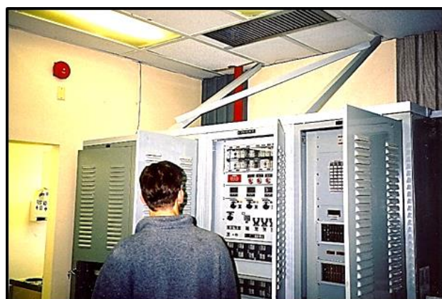
Earthquake bracing at John Hart powerhouse.
