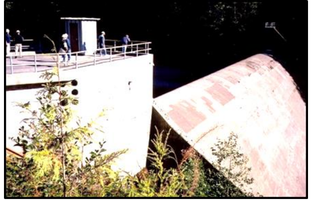
Intake structure and weir spillway.
