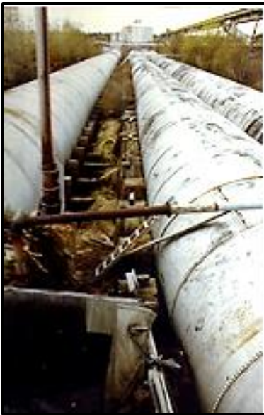
View of cracked concrete saddle.
