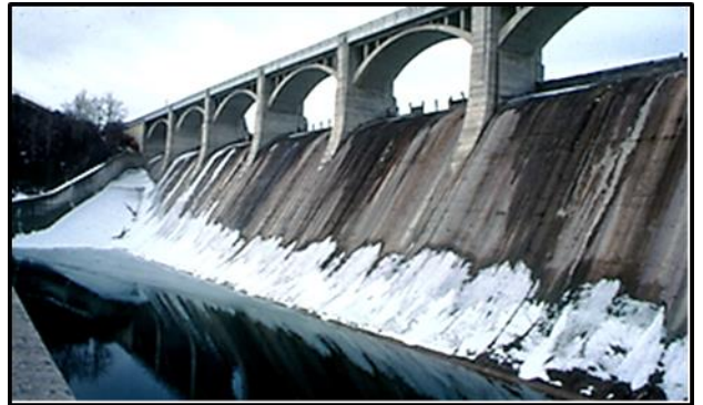
Downstream view of spillway. Note stoplogs on crest and difficult operation.
