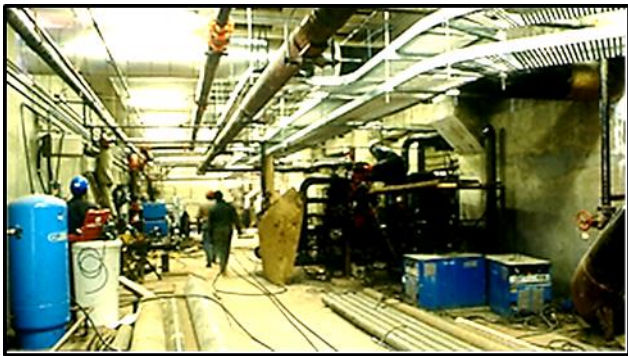
Powerhouse piping gallery during installation work.
