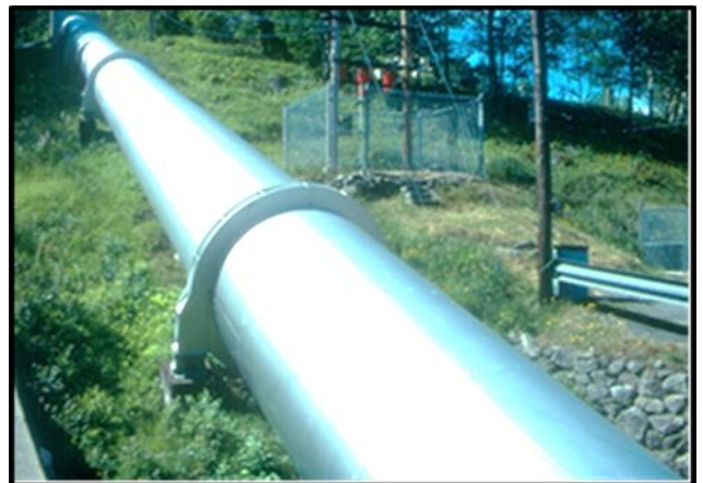
Penstock at the Gulch 6MW powerplant built in 1952.
