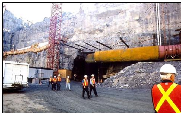
Tunnel adit at powerhouse.
