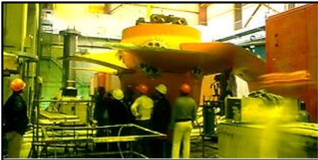
Kaplan turbine and shaft awaiting installation.
