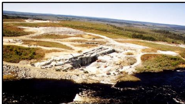
Aerial view of diversion tunnel inlet excavation.
