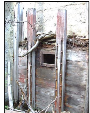
Remains of intake gate at tunnel – Note small filling gate. Source – Virtual Museum.
