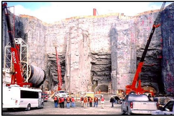
Intake excavation completed. Tunnel form on left.
