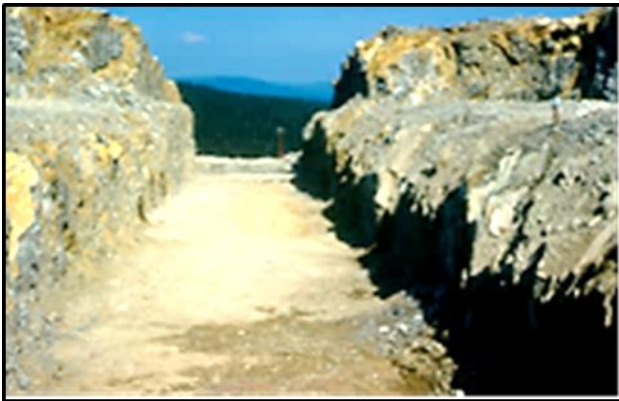
Bathtub spillway excavation.
