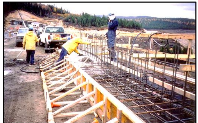
Concrete being poured into parapet wall base slab
