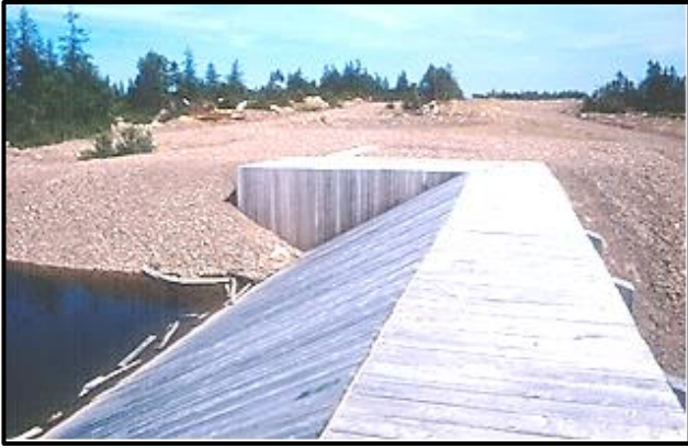
Timber crib emergency spillway.
