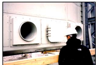
Low level valves in gate bottom.
