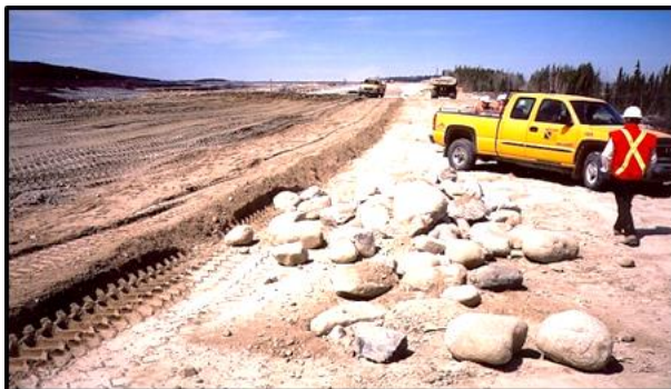
Above – Construction of Dyke LE-14. Below, boulders removed by a rock rake.
