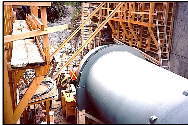
Ring girder support just before HB valve.
