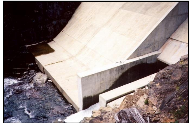
Temporary diversion outlet in weir spillway.
