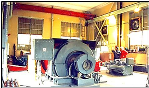
Powerhouse and generator, governor on right. Operator with Bert Budgell.
