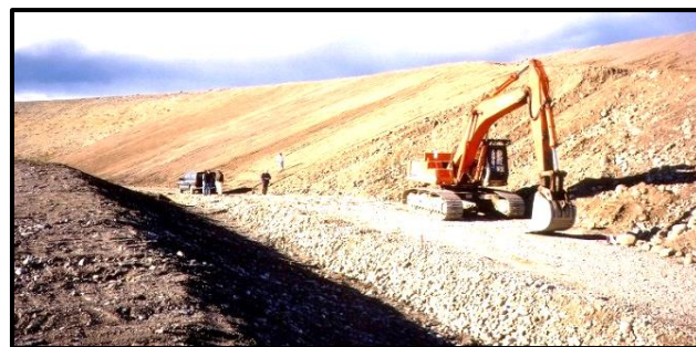
Adding fill to downstream slope at GF-8. Note smoothness of finished slope – excellent work!
