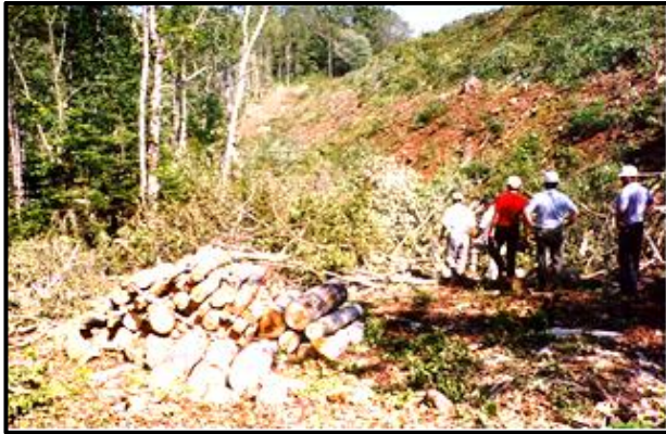
Cleared downstream slope at Lumsden Dam.
