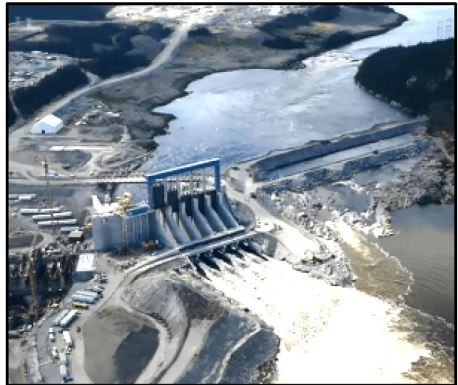
Downstream view, spillway and cofferdam.
