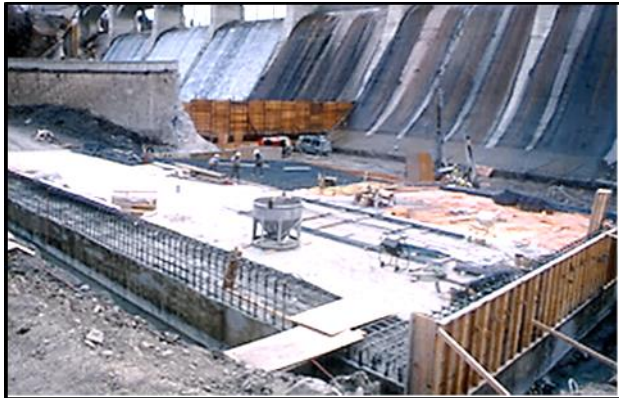
Concreting new spillway stilling basin.
