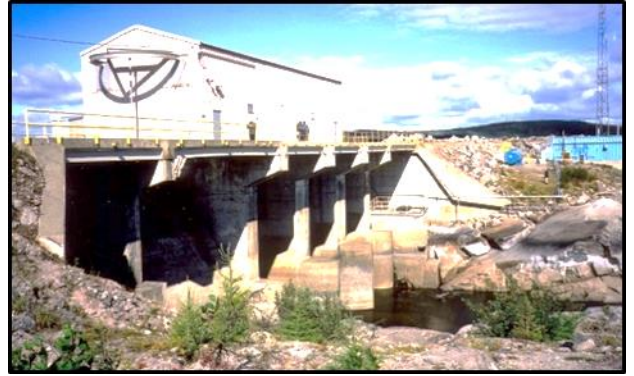
Flow control structure from right abutment. Note monorail for hoist turning around outside building.
