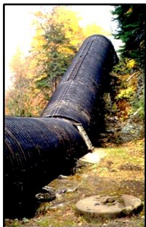
Wood stave pipe to Hydro-Fraser powerhouse.
