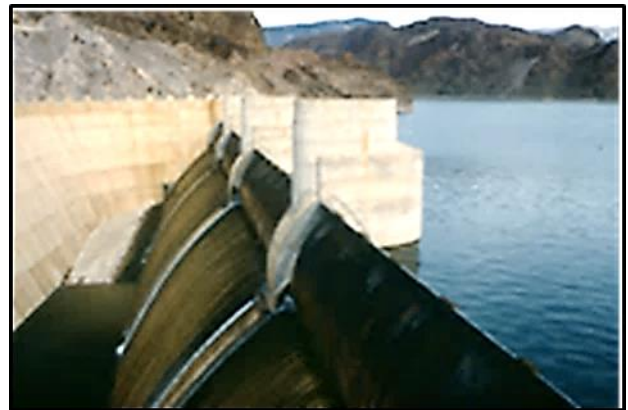
One of two side channel spillways.
