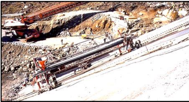
Slip-form for concrete face.
