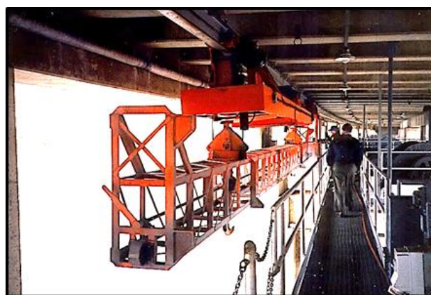
Monorail hoist for Tainter gate stoplogs.
