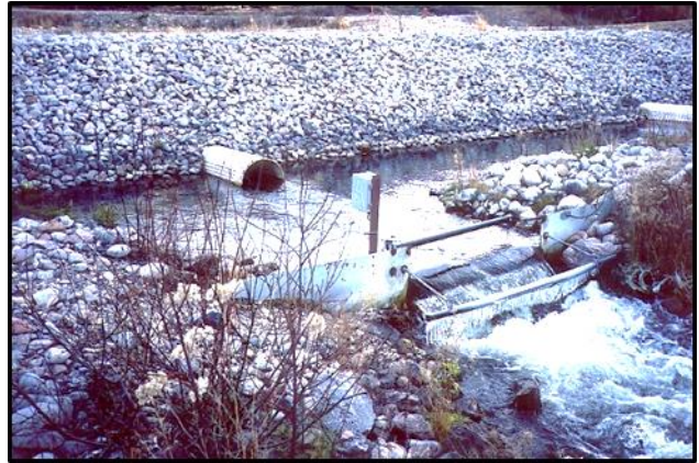
Seepage at monitoring weir below old dam.
