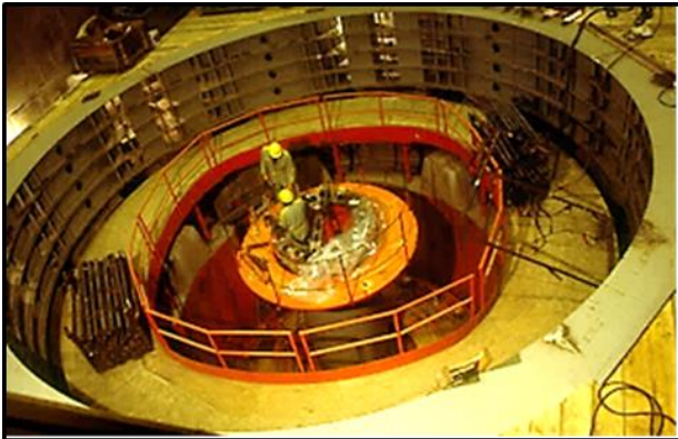
View looking down into generator stator frame, no poles attached. Machinists working on turbine shaft.
