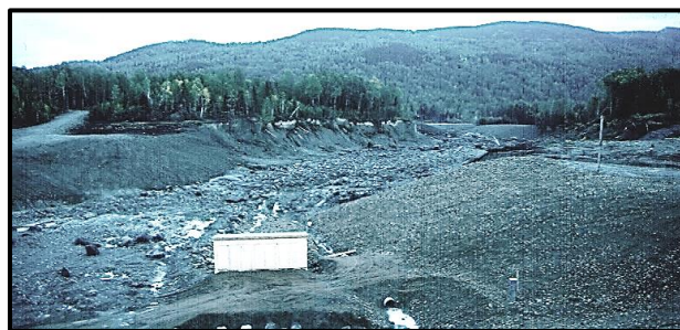
View of dam breach. New weir added downstream.
