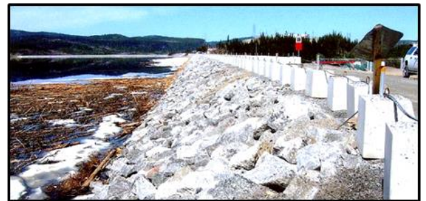
Completed main dam upstream face.
