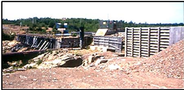
Intake with timber crib flanking dams.
