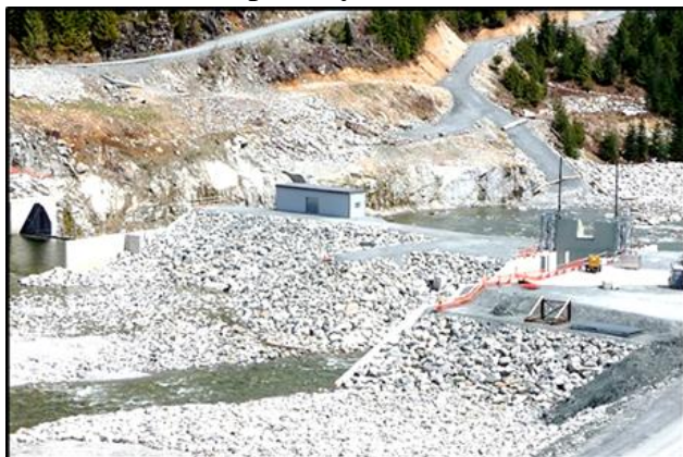
Spillway, dam and intake. Building has hydraulic hoist servo pumps for spillway.
