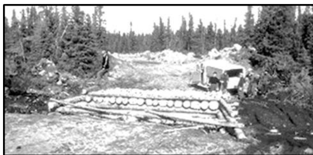
Timber culvert.
