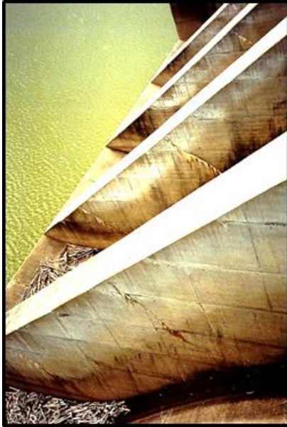
View of 45-degree cracks in spillway piers.
