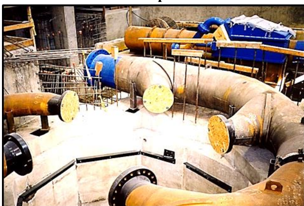
Distributor for 5-jet impulse unit.
