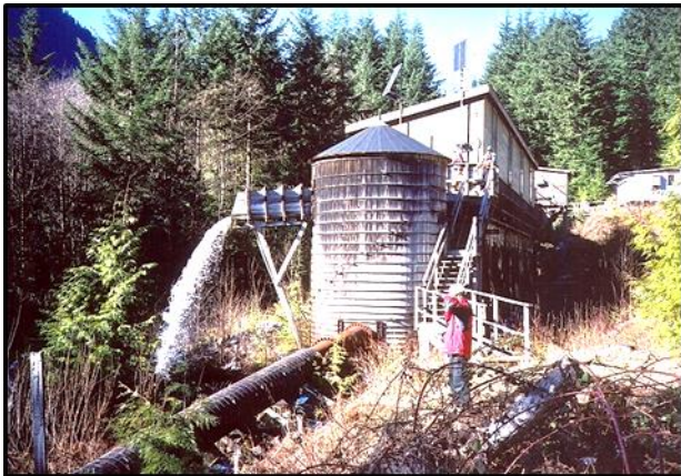
Cedar Creek screen house and tank – note penstock.
