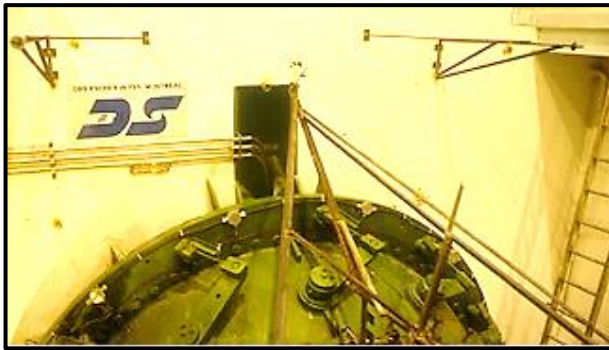
Brackets attached to intake wall for plumb-bobs.
