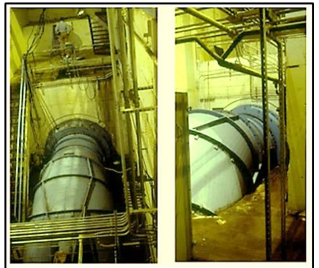
Two views of tube turbine. Note oil piping.
