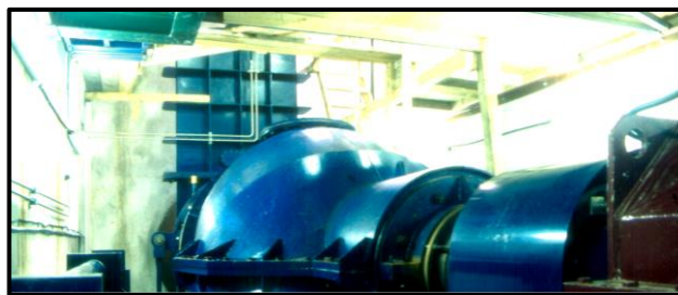
View of turbine. Note abrupt right-angle bend immediately upstream of turbine.
