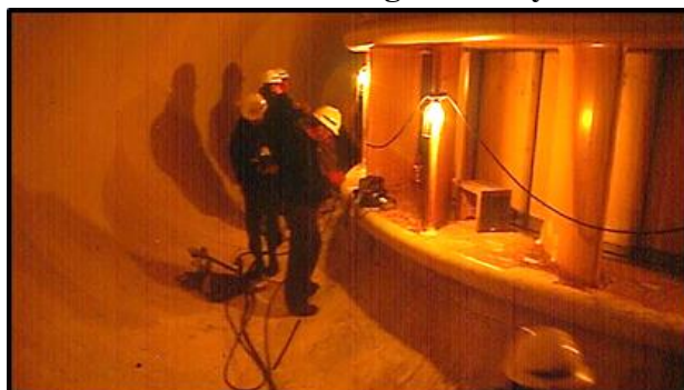
Inside turbine steel spiral casing.
