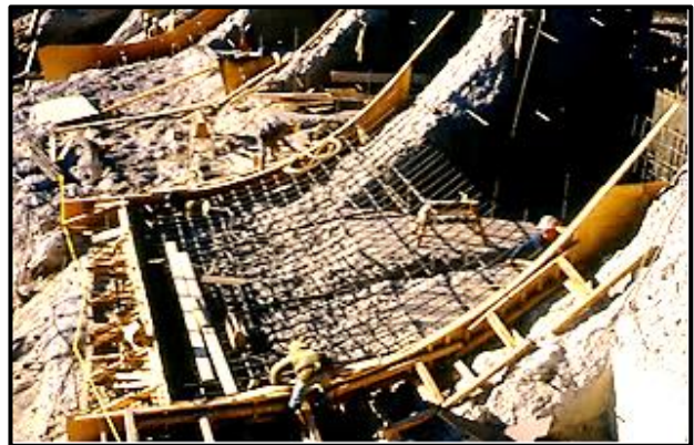
Reinforcing for flip bucket – main spillway.
