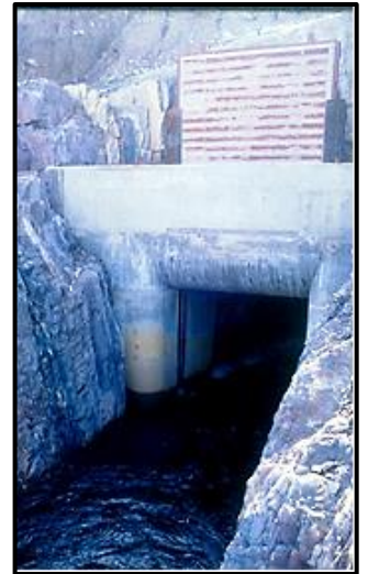
Diversion tunnel intake with concrete-steel gate above.
