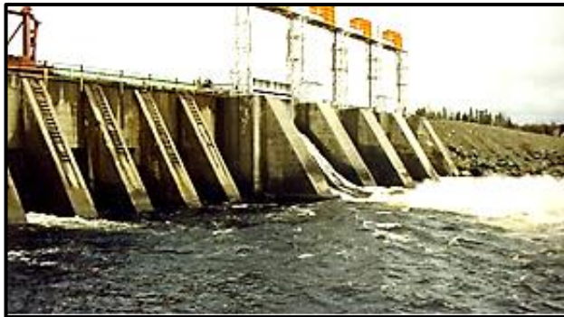
Low level sluices and 4 spillway gates.
