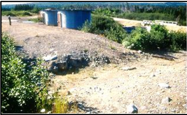
South Twin Dam with trench on crest.
