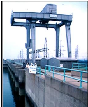
Intake gantry crane
