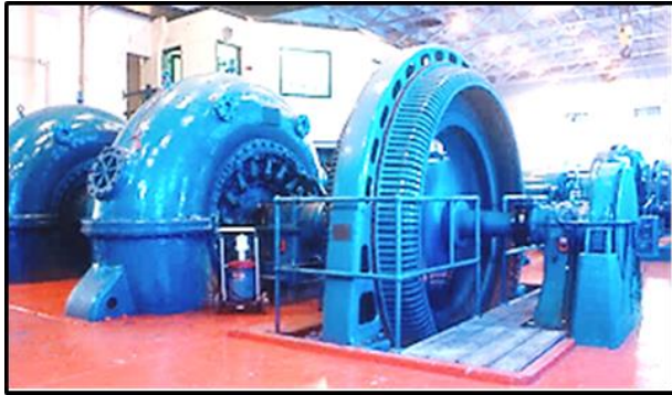
Powerhouse containing 4 horizontal axis Francis units.
