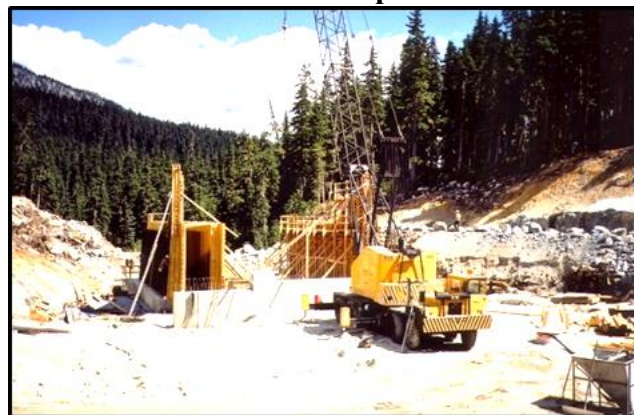
Headpond dam, formwork for spillway.
