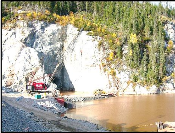
Placing cofferdam at diversion tunnel outlet.
