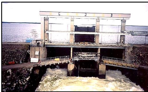
Lobstick Gate #2 channel repaired. Other gates will be closed to permit removal of middle gate stoplogs in calm water.
