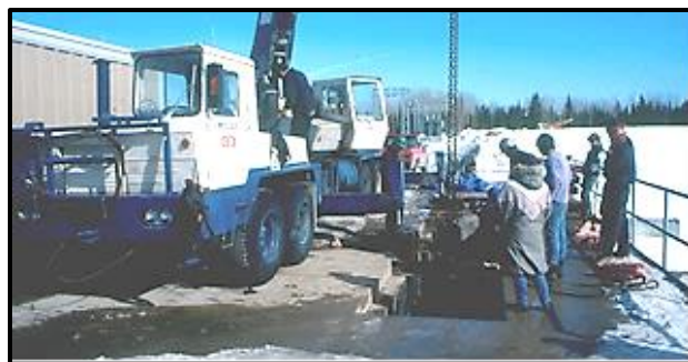
Lifting intake gate with mobile crane.
