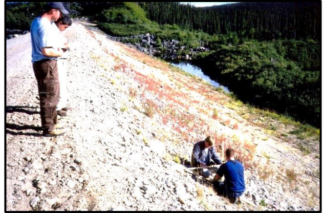
1.6:1 slope on GL-8 near left abutment. The reddish vegetation is "Labrador tea".
