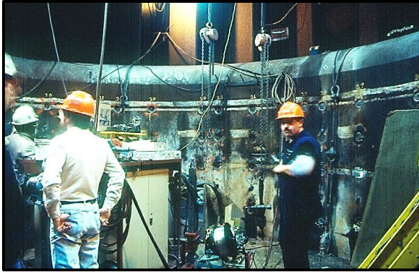
Anchoring turbine throat ring.
