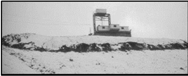
View of earth starting to slide off, below intake.
