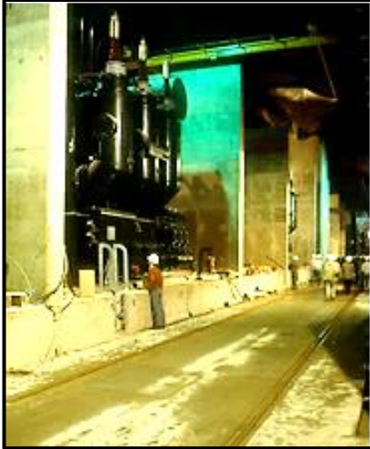
View of transformers in draft tube gallery.
