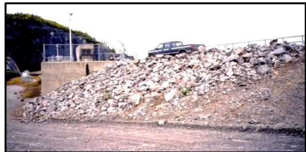
Rip-rap on downstream slope of dyke.
