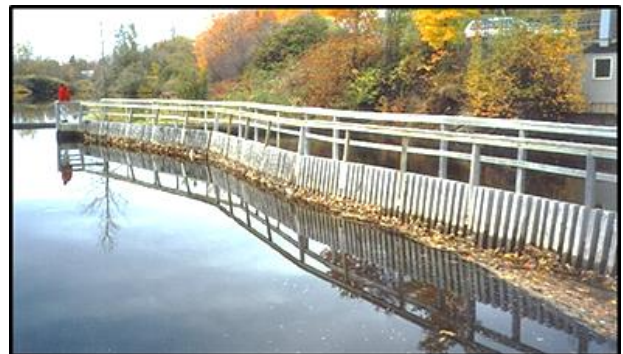
Timber trashracks at entrance to intake channel.
