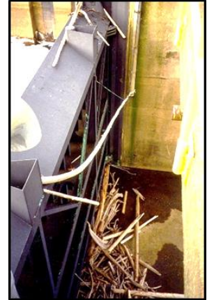
Looking down back of gates – note flow splitters.
