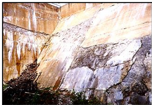
View of deterioration at junction of intake with dam.
