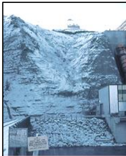
View of earth slide downstream of intake.
