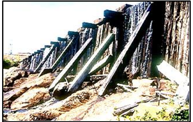
Props on timber crib weir dam at intake.
