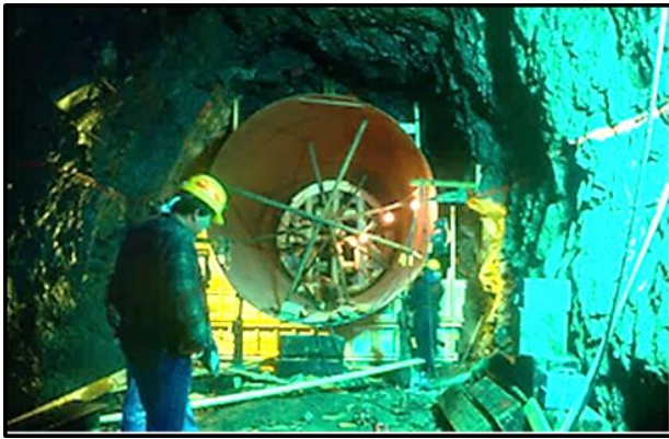
Start of penstock installation within tunnel.
