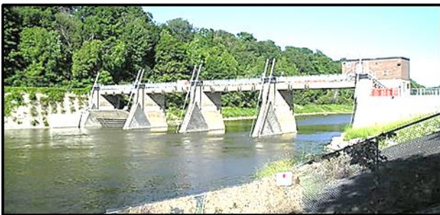
Downstream view of four new gates with hydraulic hoists – note jammed gate at left.
