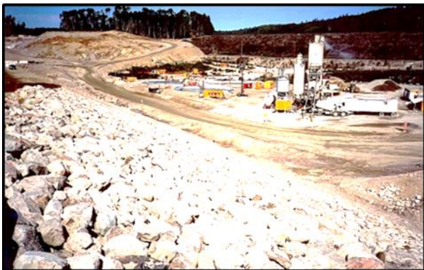
Carefully placed rip-rap on upstream face.
