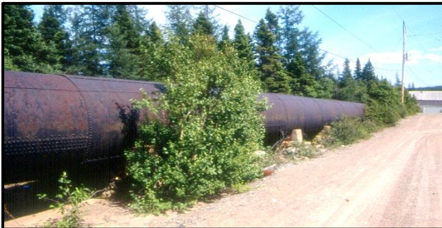
Penstock along the side of the access road to powerhouse
