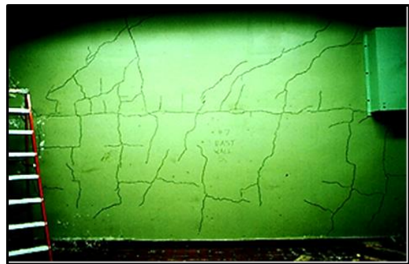
Mapwork cracking on a wall.
