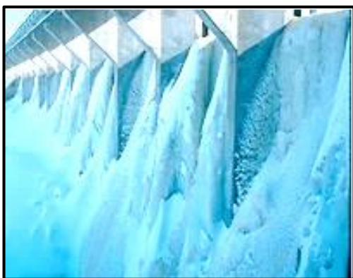
Downstream view of iced-in gates.
