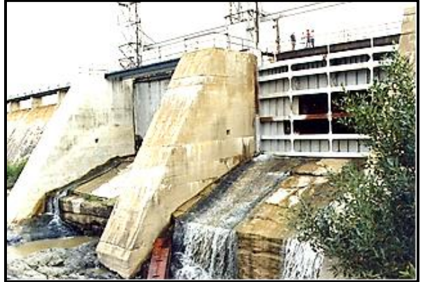
Two spillway gates. Note missing downstream panels.
