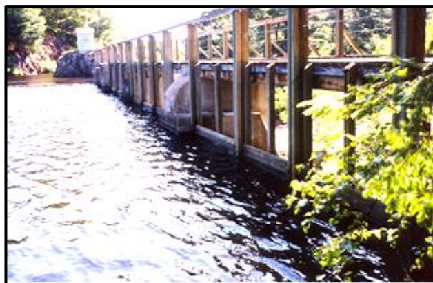
White Rock stoplog weir spillway, upstream view.
