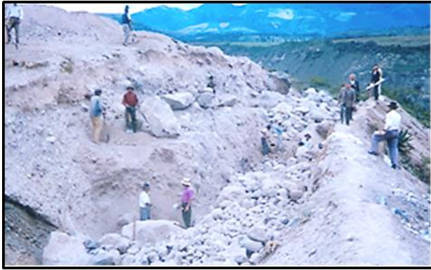
Excavating the intake canal.
