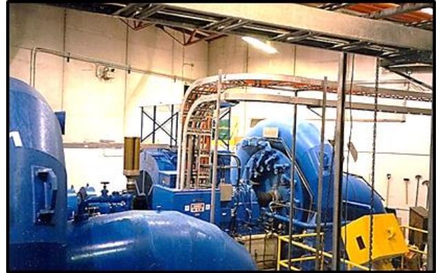
Powerhouse interior, turbines – note no crane.
