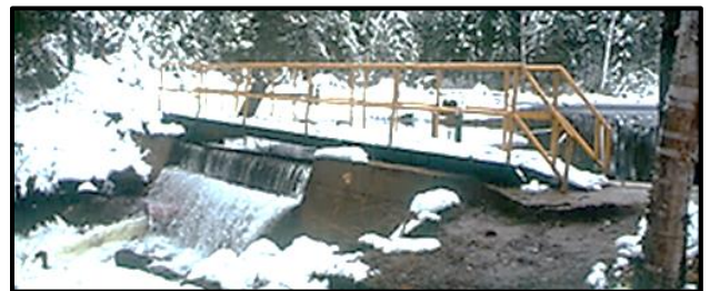
Upstream and downstream views of weir and intake screen. There is an uncontrolled low level outlet for compensation water.
