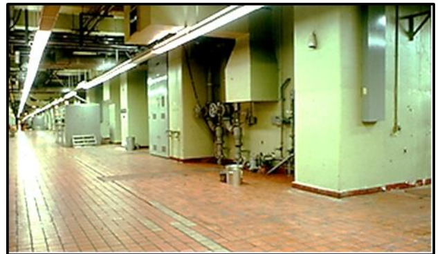
Floor at El. 174. Grey tiles replaced old cracked tiles.
