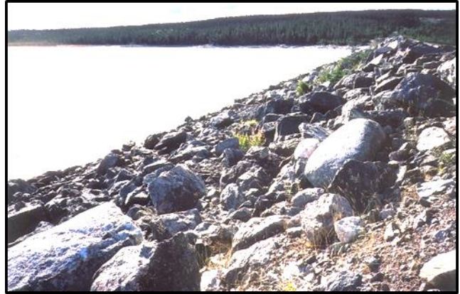
View of missing rip-rap at nose on Pudops Dam.
