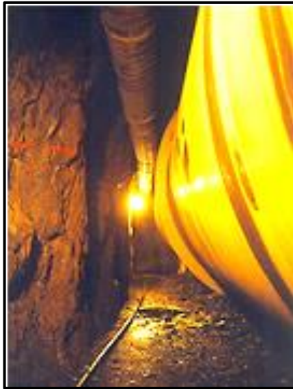
Start of penstock installation within tunnel.
