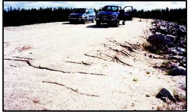
Rain erosion of crest in low area.
