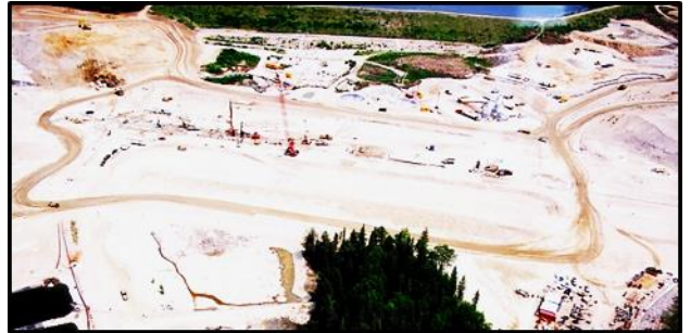
Cut-off wall during construction. Old dam at top of photo.
