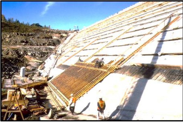
Horizontal planks are work platforms for filling kerb gaps with concrete. Workers are placing horizontal re-bars.
