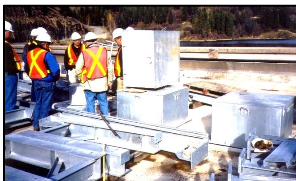
Completed anchors with covers.
