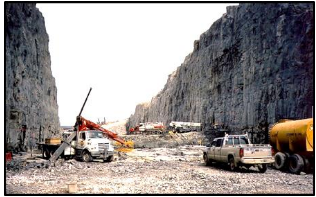
Looking upstream in spillway chute excavation.
