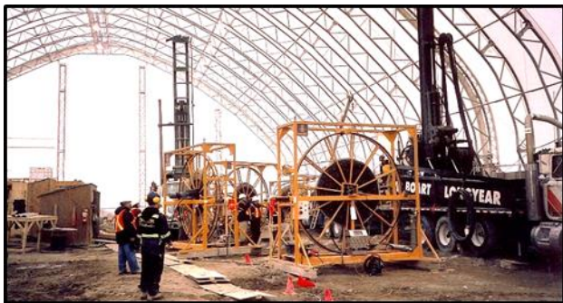
Hoarding over cut-off wall grouting work on main dam during winter.
