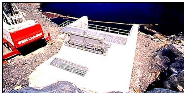
Intake with headgate dogged open.
