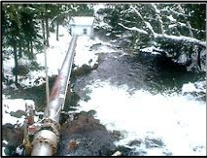
Penstock and shut-off valve.
