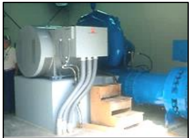
Small Francis turbine in second powerhouse.
