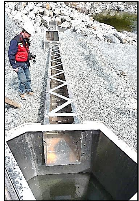
View of steel fish ladder.
