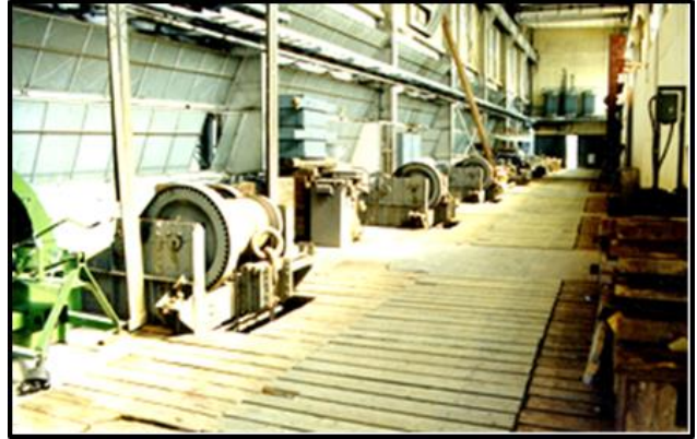
Headgate hoist house. Gates - trigger close, crane open.
