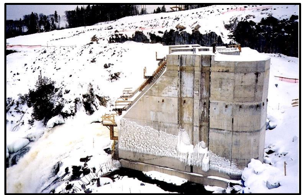
New spillway pier.
