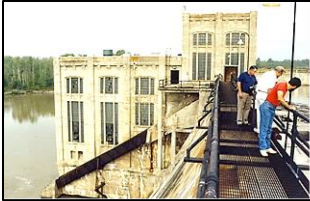
Log chute at end of Twin Falls powerhouse.
