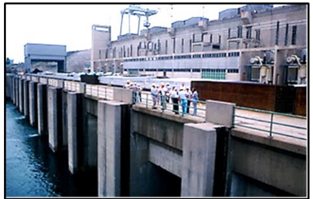
View of pump-turbine "draft tube" deck and powerhouse roof. Intake gantry at top.
