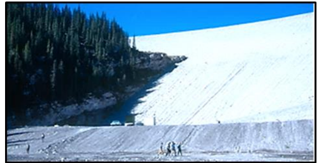
Inspecting downstream toe of dam for seepage. Note large toe berm.
