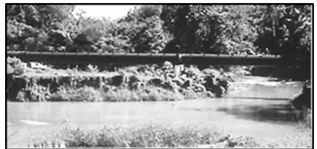
Steel pipe bridge over Maggotty River.
