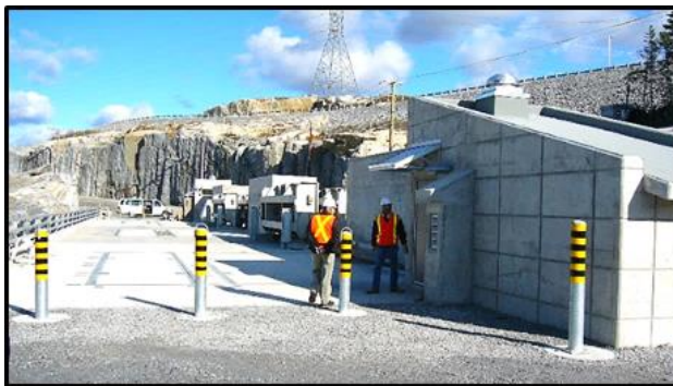
Intake deck with air vent housings.
