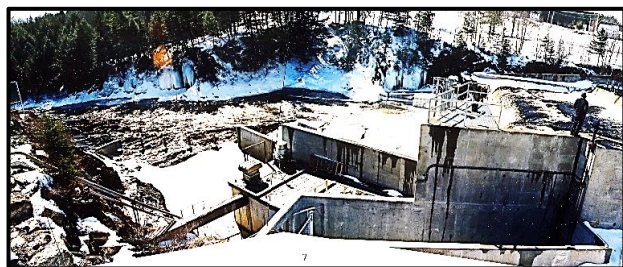
Panorama – powerhouse, by-pass sluice and tailrace.
