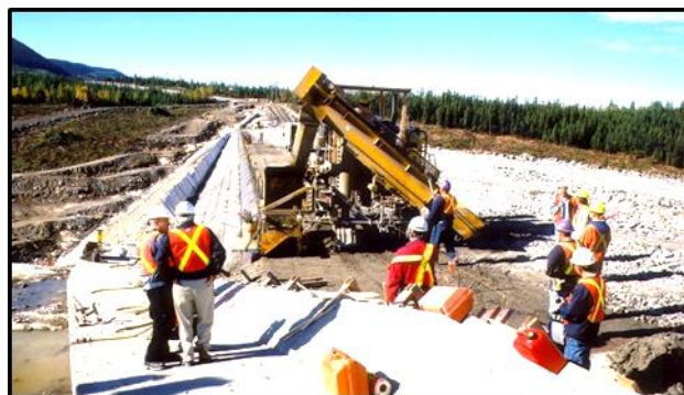
Machine placing kerb in horizontal strips at top, along face of the rock fill.
