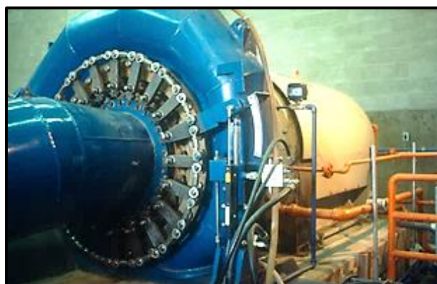
Wicket gate servomotor.
