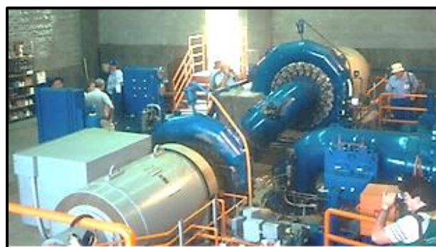
Francis turbines of 1.0 and 2.0MW capacity.
