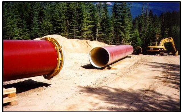
Penstock pipes down to powerhouse.
