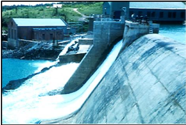
Two views of downstream face, repaired concrete.
