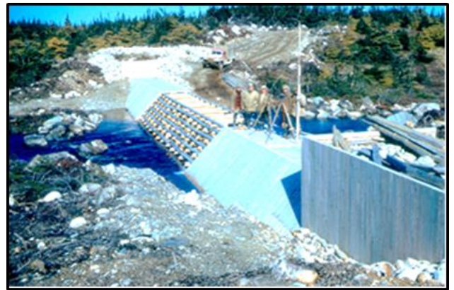
Almost complete Fourth River timber crib dam.
