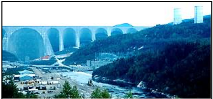
East bank, note surge tanks and initial powerhouse.
