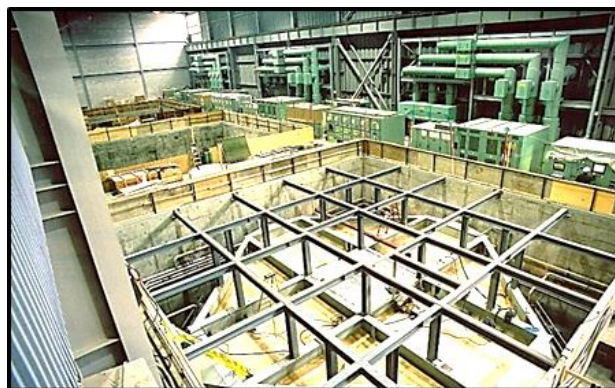
Generator casing assembly.
