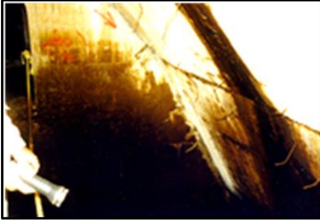
Interior of Ambursen dam spillway. Sloping face is upstream concrete face on dam. Dark portion is seepage at joints.
