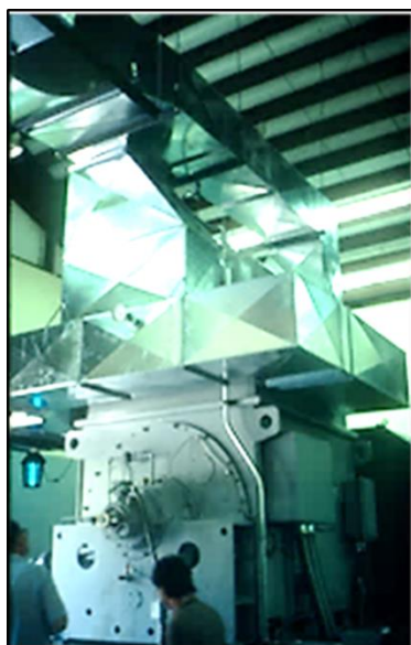
Cooling air ductwork above generator.
