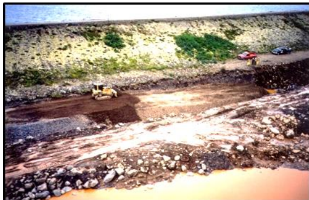
GL-21 work. Dark green vegetation could indicate seepage.
