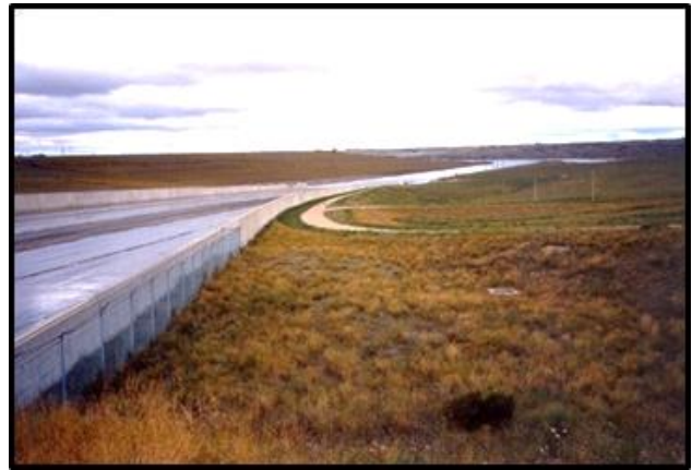
View looking down dam slope at spillway chute. Note extremely flat downstream slope on dam.
