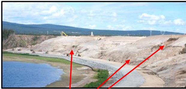
Reshaping work on the upstream face. Note slips on face.
