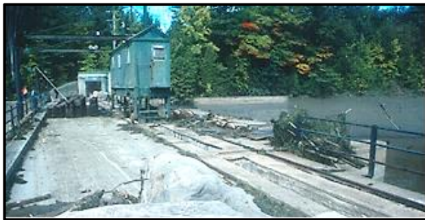
Debris on dam crest after 0.6m overflow.
