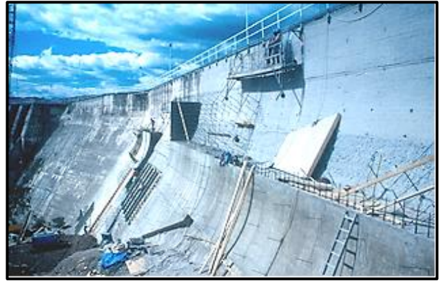
Adding concrete to downstream face of dam.
