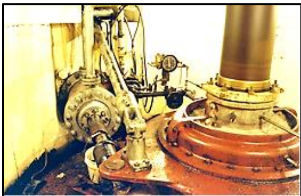
Turbine servomotor.
