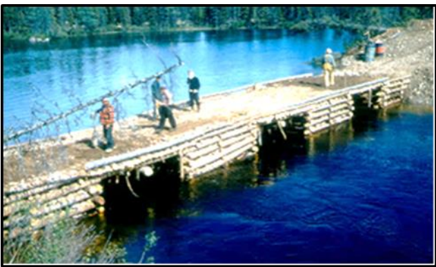
Timber crib bridge.
