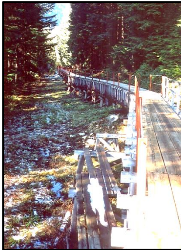
Intake sill and start of wood flume.
