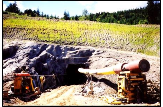
Tunnel adit near intake structure.
