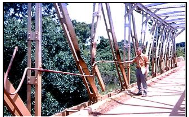
George inspecting bridge – note bent and broken truss steelwork.
