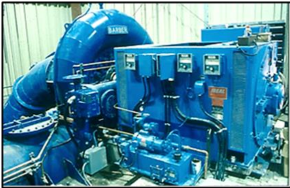
New Barber unit, induction generator.
