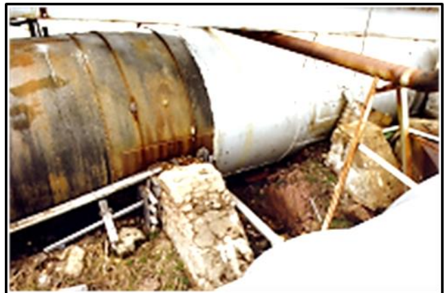
View of patched penstock at saddles.
