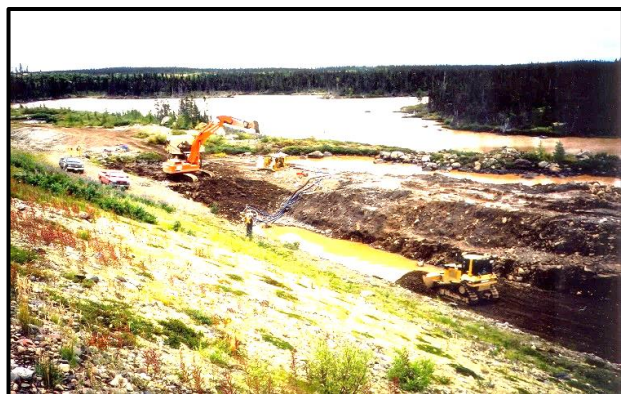
Adding drains and toe berm at GL-21.
