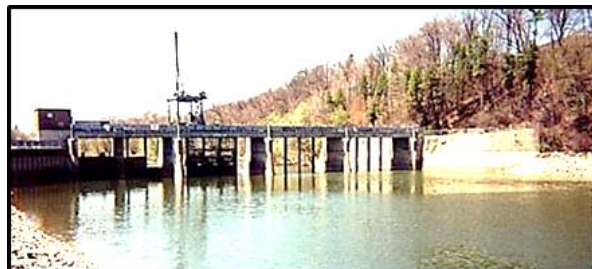
As re-built in 1929. Stoplogs being removed. Source – www.thamesriver.on.ca
