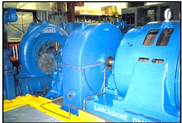
Horizontal shaft Francis turbine, with large flywheel in middle for isolated operation.
