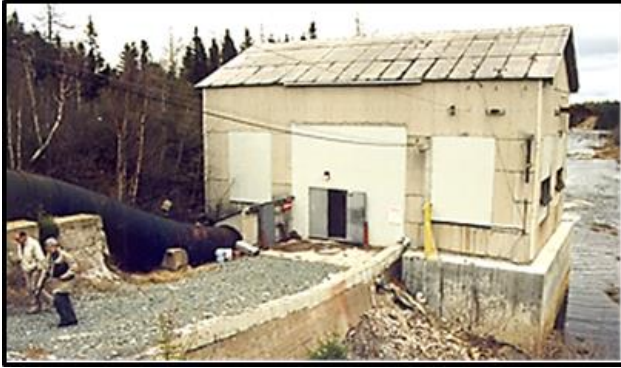
Powerhouse with upstream windows covered as protection from vandalism.
