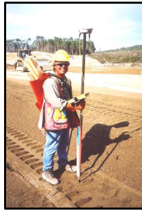
Left – surveyor with GPS and computer on staff. Knapsack full of stakes to place at intersection of material sections.
