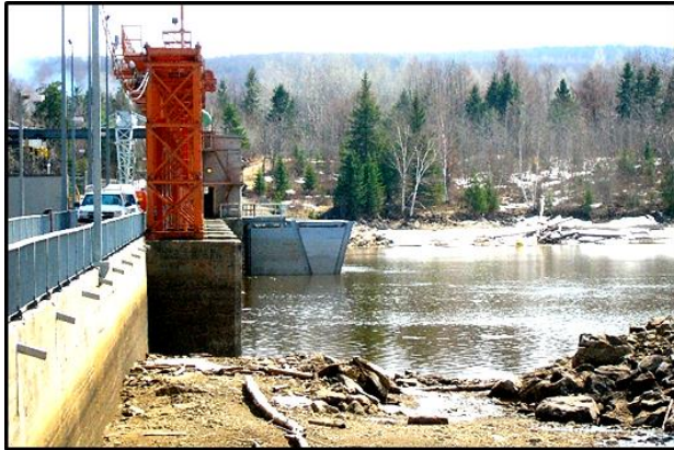
View of steel box syphon intake.
