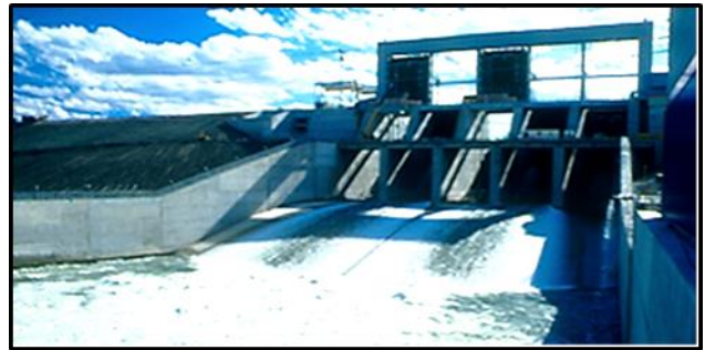
5-gated spillway, passing diversion flow.
