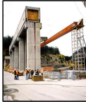
Steel towers being installed, hoists now on deck.
