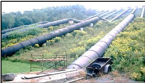
DeCue old riveted steel penstocks.
