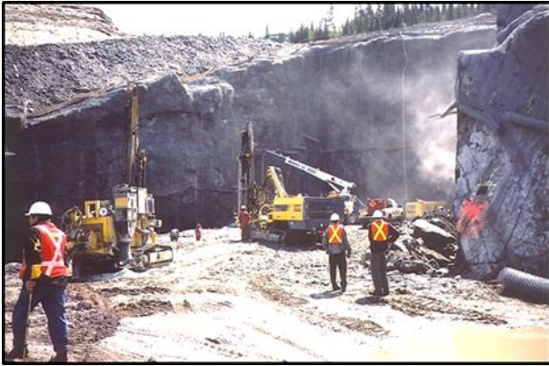
Inlet channel for diversion tunnel.
