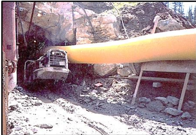
Very tight fit for low pressure tunnel excavation equipment.
