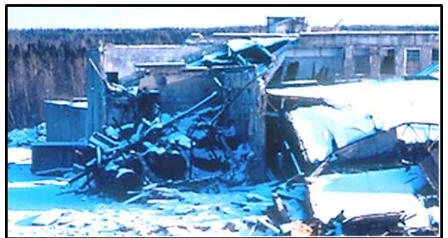
View of washed out wood room and no dam.
