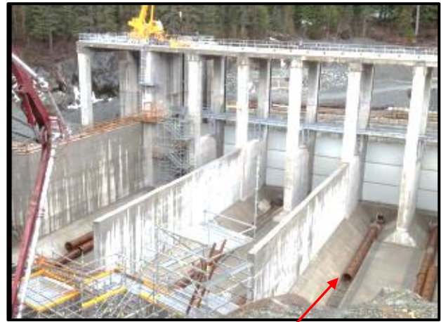
Intake, looking upstream. Note sand trap pipes.
