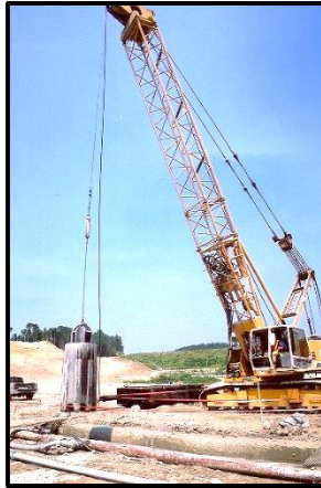
Chisel used to cut through boulders and into rock foundation.
