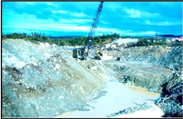
1.2m 3 dragline excavating canal from 4th pond.
