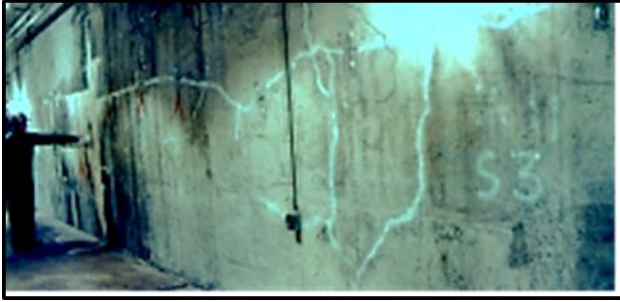
Cracking on casing El. 143, outside wall.
