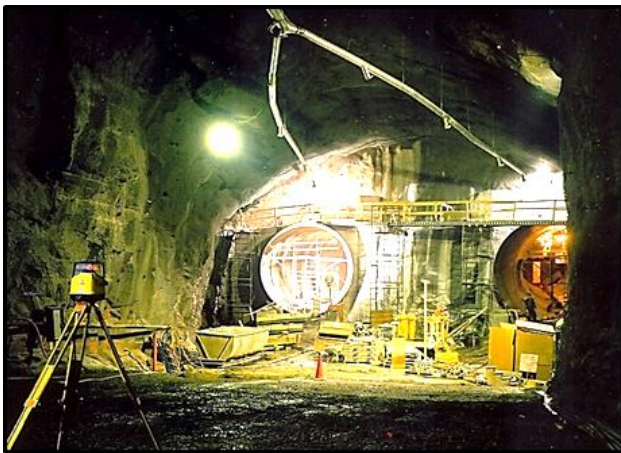
Power tunnel at powerhouse bifurcation.
