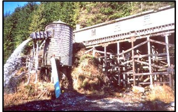
Mill Creek tank where surplus waters removed. Screening room on right.
