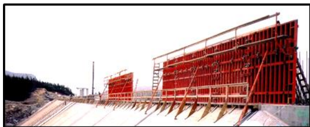
Formwork for high parapet wall on main dam crest. Note spillway gate hoist structure at far left on side dam.
