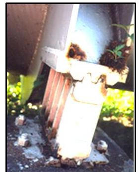
Rocker support for ring girder on Gulch penstock.
