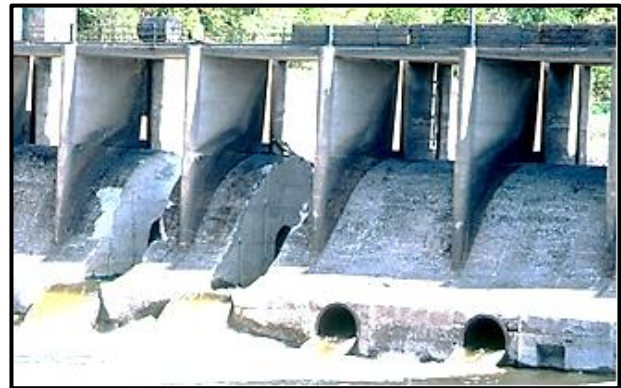
Cut-down ogees and low level outlets discharging.
