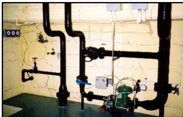
Powerhouse turbine floor, mapwork cracking outlined with pen.
