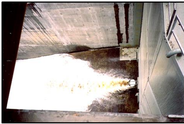
Testing one of the gate valves.
