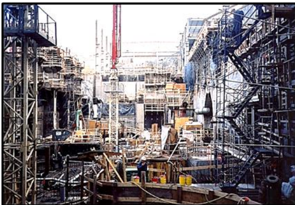
View across powerhouse – penstock tunnels on right.
