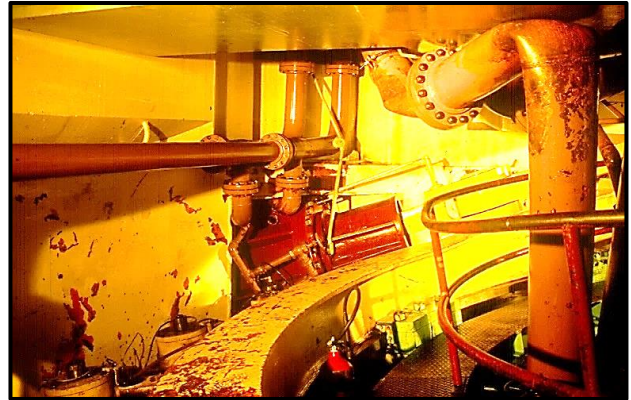
Same view Unit #1. Damaged. Note angled turbine cover and angled ruptured red turbine servomotor, which was full of oil.
