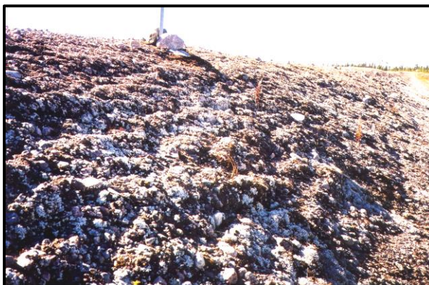
Surface cracking and slipping at GR-10
