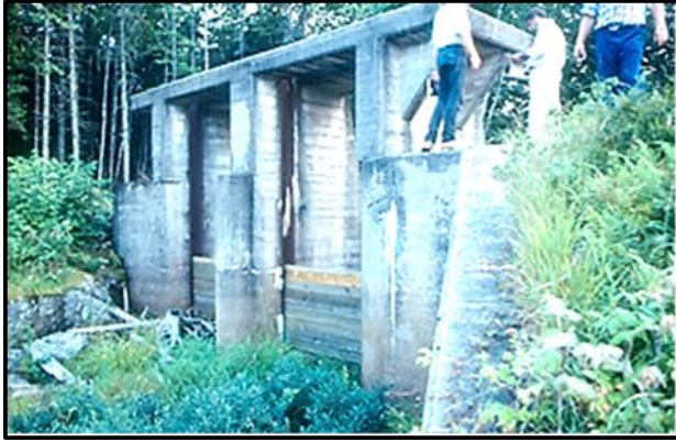
Concrete spillway with stoplog control at Paradise Dam.
