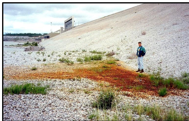
Seepage at downstream toe.
