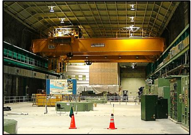
Completed generator floor and two 205 ton cranes.
