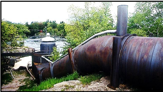
Steel penstock down to powerhouse.
