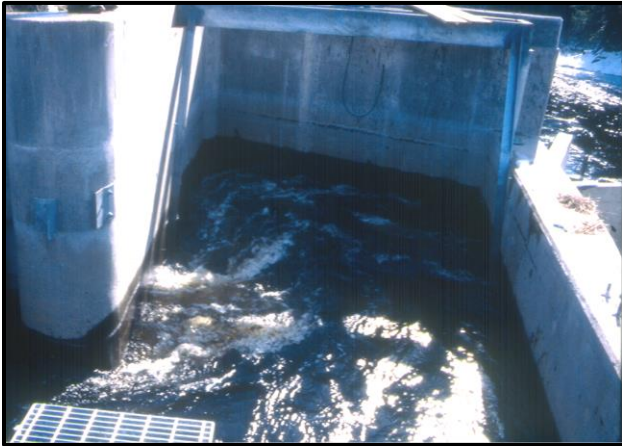
Large vortex beside pier at maximum power output.
