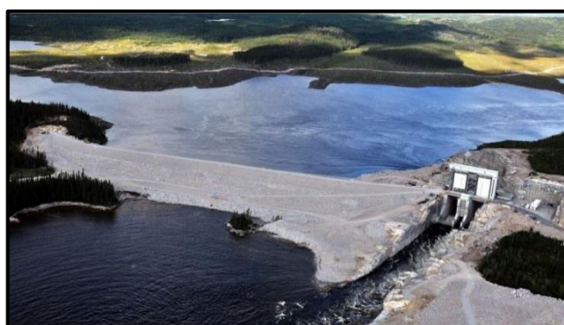
View of Rupert Spillway, completed. Hoist access to gate hoist moved to opposite end. Source – CBC News.
