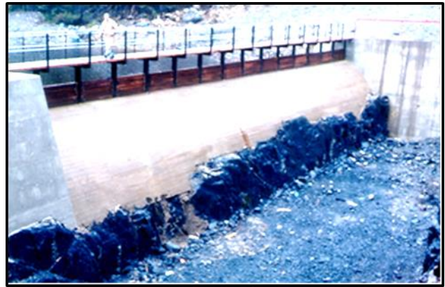
Gull Pond dam with stoplog control.
