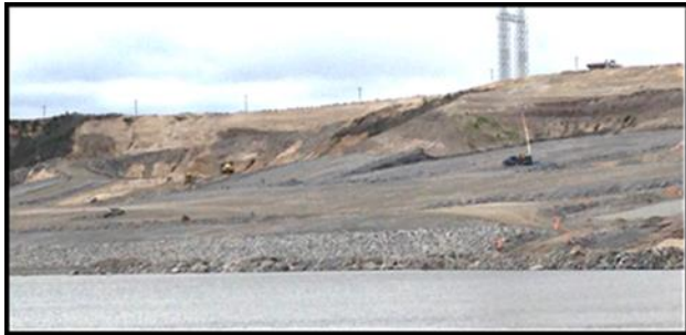
Re-shaping work on the downstream face. August 2016.
