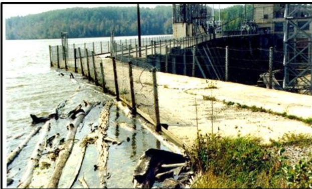
Oops – no freeboard! Fence to prevent driftwood flowing over dam during a storm.
