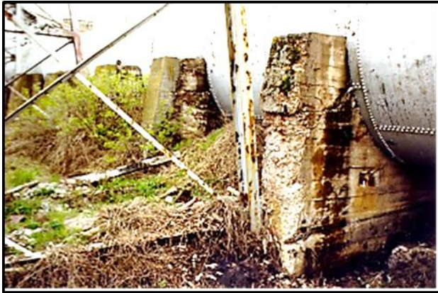
View of cracked concrete saddle.
