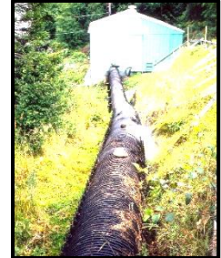
Below – leaky pipe near powerhouse.
