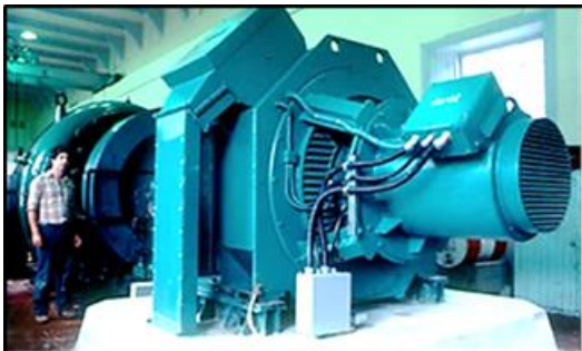
New generator and exciter.
