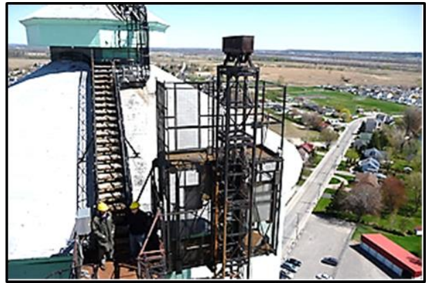
Rack-climbing elevator at top of tank.
