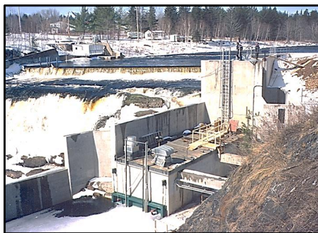
View of powerhouse and intake shaft. The two men are standing on the intake deck.
