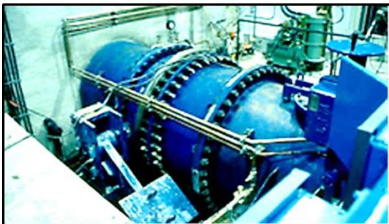
Turbine inlet valve.
