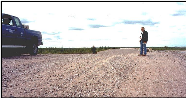
Below – Wavy dam crest on discontinuous permafrost foundation.
