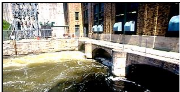
Unit #1 tailrace flow at full load.
