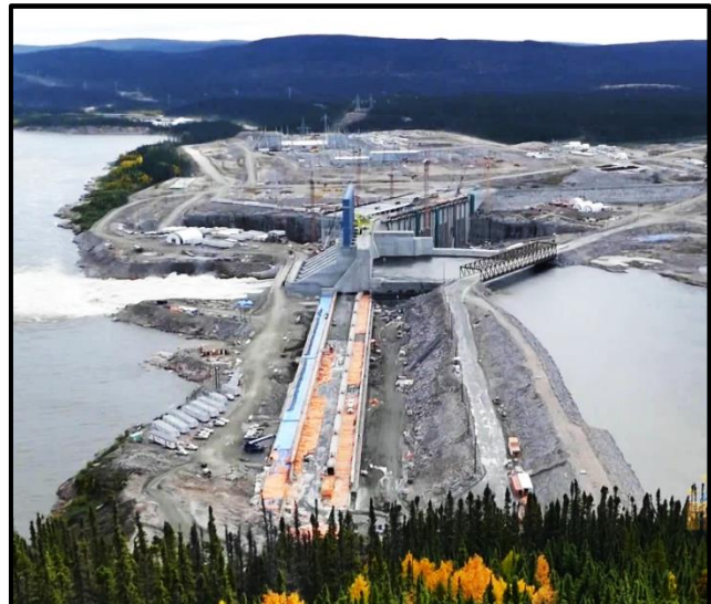
RCC dam construction.
