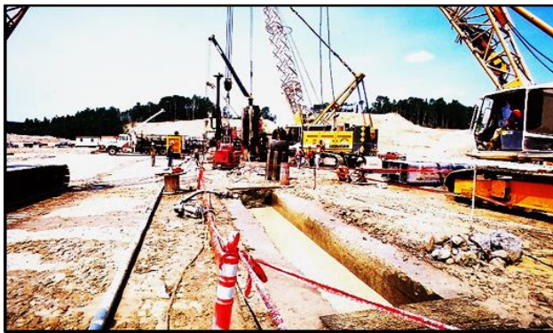
Excavation of a panel. Note similarity to Peribonka.
