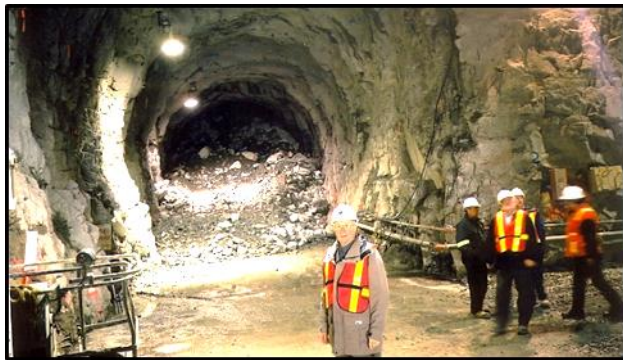
At access cross-tunnel junction, for penstock excavation near powerhouse.
