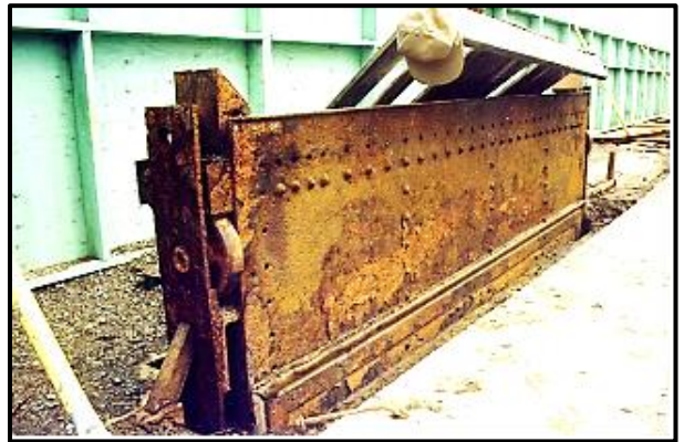
Rusty low level sluice gate.
