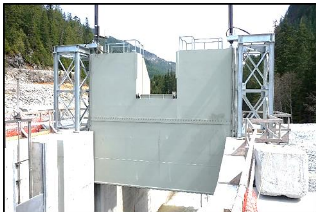
Spillway gate with small compensation flow gate.
