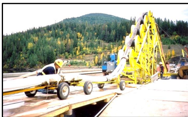
Roller jig used to turn anchors to vertical.
