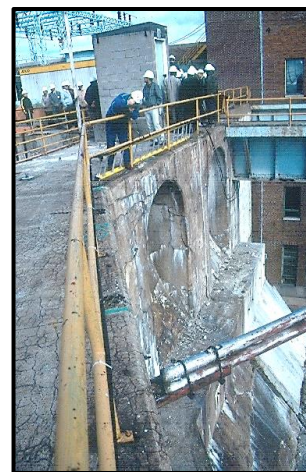
Cracks from AAR in abutment and an inside wall.
