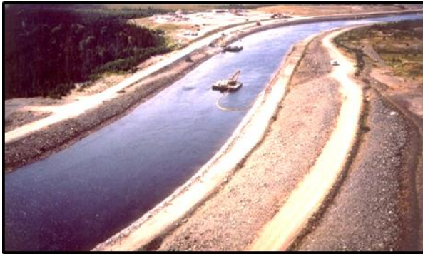
Salmon Canal – slope by hill being flattened.
