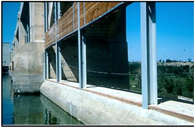
Detailed view of wood gate guides.
