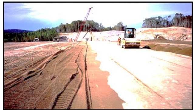
Compacting core material on dam. Cut-off completed.
