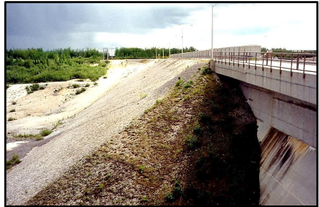
A well-graded downstream slope.
