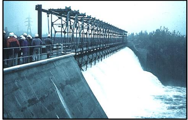
New spillway gates and monorail hoist.
