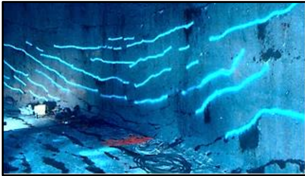
Cracks sloping down to middle in semi-spiral casing.
