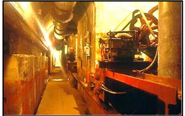
Drainage gallery and low level outlet operator.
