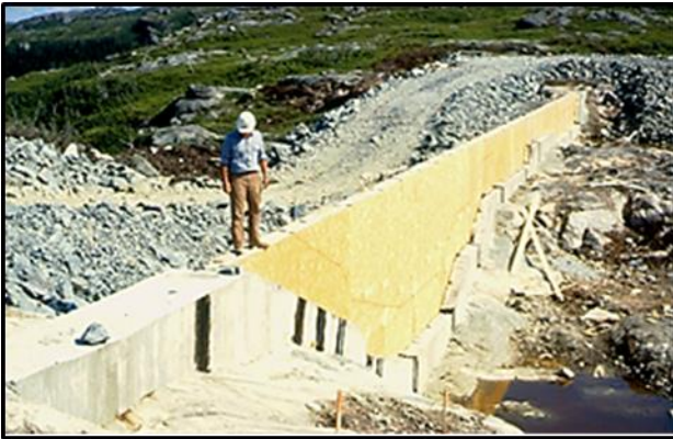
Concrete core wall in a small side dam.
