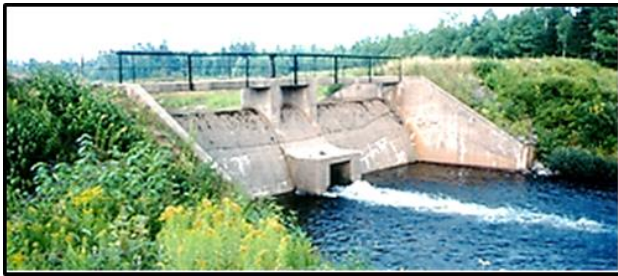
Concrete weir and low level outlet at Paradise Reservoir.
