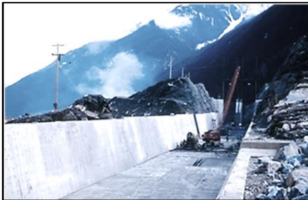
Looking up the spillway chute.
