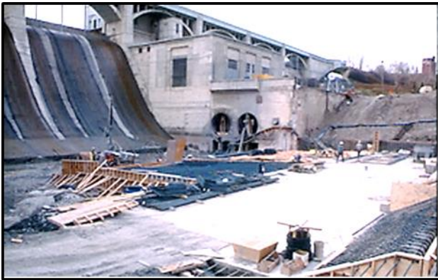
View towards left abutment – new stilling basin. Two pipes are low level outlets.
