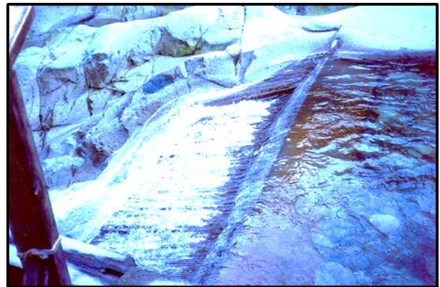
Intake with sloping bottom trashracks.
