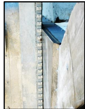
Gate seal jammed against right pier.
