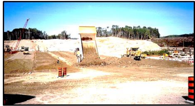
Placing embankment material.
