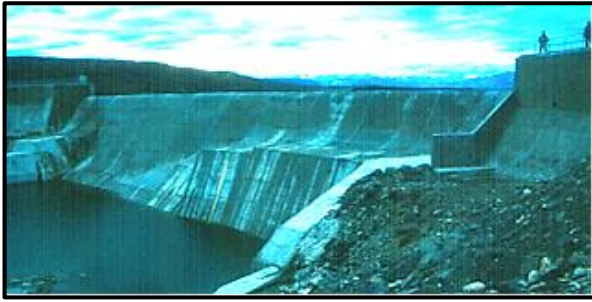
Completed auxiliary spillway weir.
