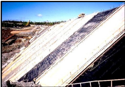
Slip-form for concrete face.
