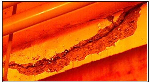
Large crack in concrete beam.
