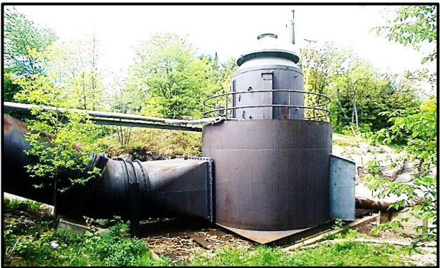
Packaged powerplant – transported to site intact.
