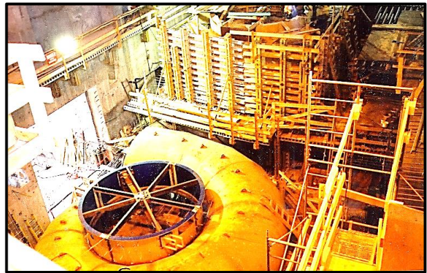
Steel spiral casing for new turbine.
