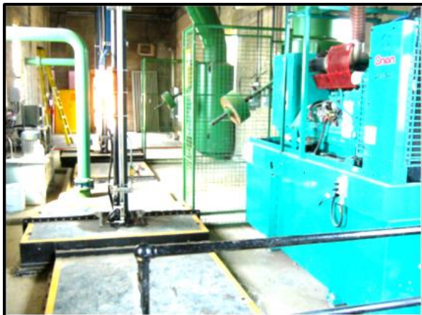
Emergency generator and intake gate hoists.
