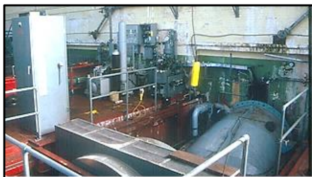
Unit #3. New hydraulic unit for gate, top left center.
