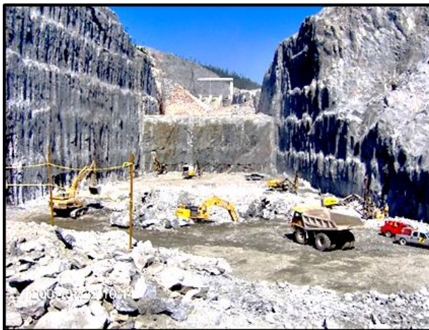
30m drop into spillway chute plunge pool excavation.
