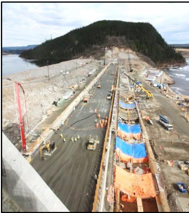
RCC dam construction across river.
