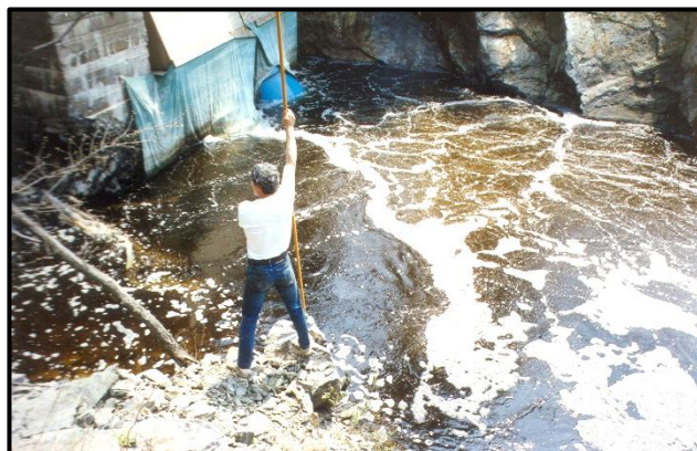
Tailrace flow. White foam indicates excessive air in the water due to the high intake velocity.
