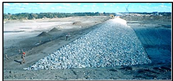
Fuse plug spillway dyke – reservoir not yet filled.
