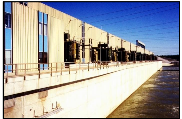
Powerhouse tailrace deck with 12 transformers.
