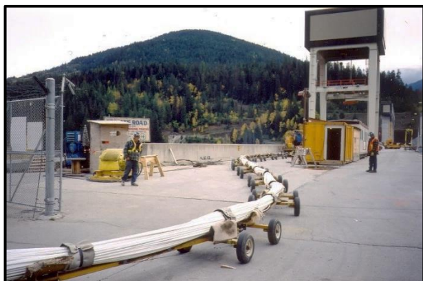
Anchor train arriving on dam.
