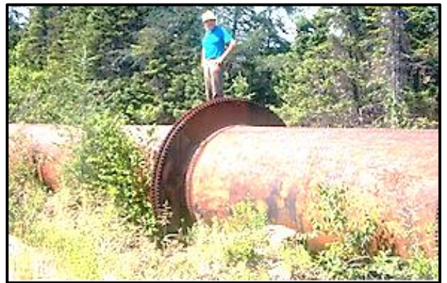
Bellows expansion joint.
