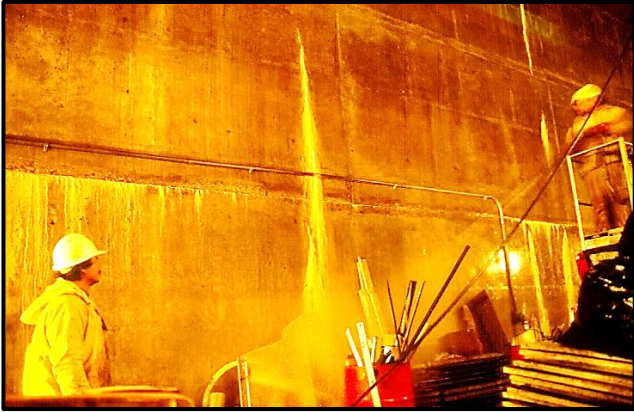
Pressure washing walls and floors to remove oil.
