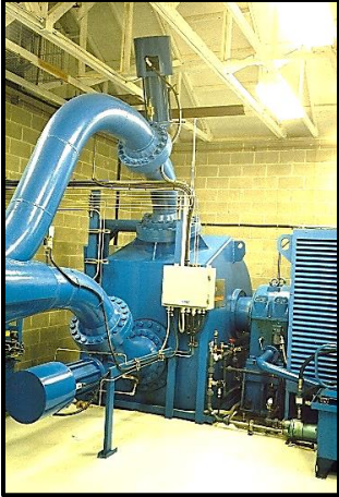
Spherical turbine inlet valve.
