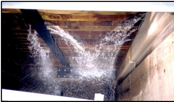
Stoplog bay with center steel column. Leakage expected to reduce when the new timber stoplogs swell.
