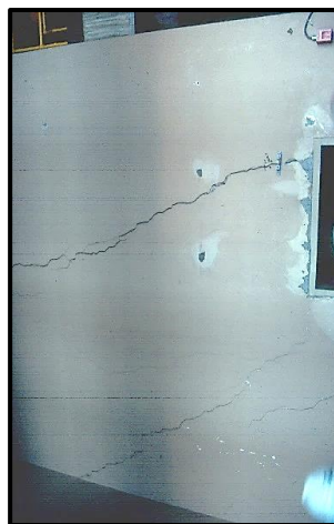
Cracks from AAR in abutment and an inside wall.
