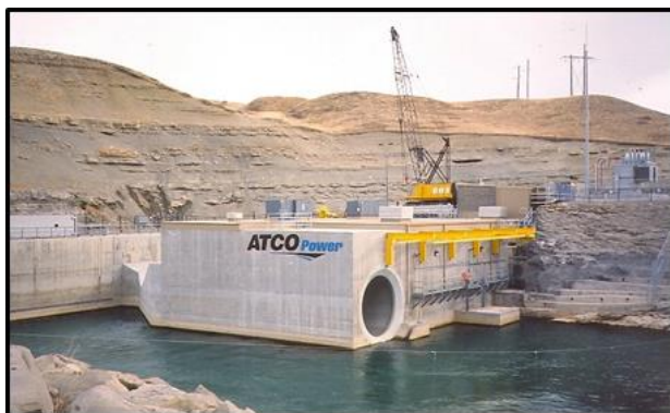
The new powerhouse. Crane about to lift out generator for repairs. Large hole in wall is relief valve outlet.
