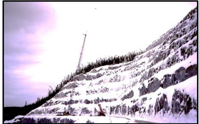
Spillway abutment excavation – crane installing wire mesh for safety.
