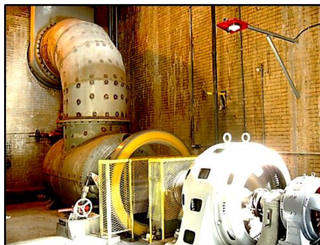
“Tin can” station service unit – operating since 1911.
