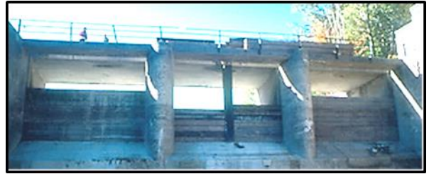
View of quick-release stoplogs, middle sluice.
