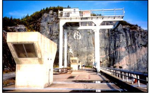
Intake deck with gantry crane. Grab for trash removal. Hoist can lift trashracks and gates to above deck. Each air vent has 2 openings.
