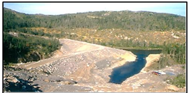
Upstream cofferdam, canal to diversion intake.
