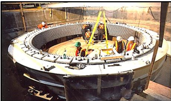
Installing 45MVA, 13.8kV generator. Speed 180rpm.
