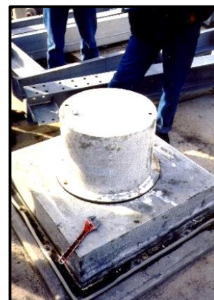
Completed anchors with covers.
