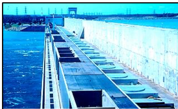
View of powerhouse roof with generator hatches.
