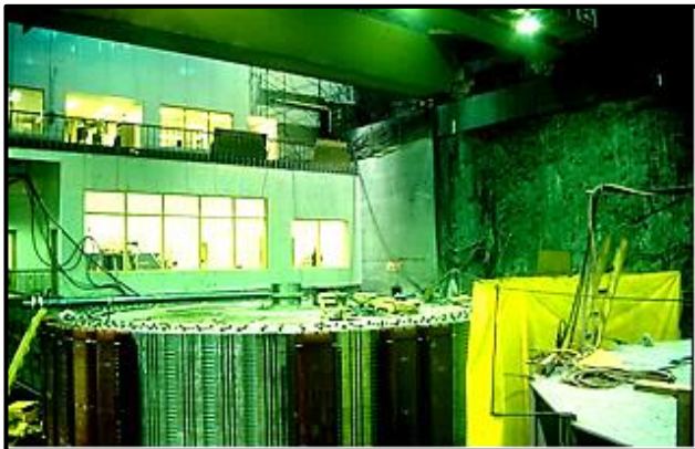
Assembly of the generator 10.4m diameter rotor.
