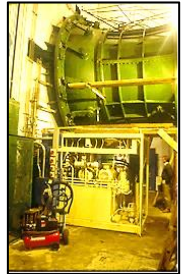
View of “S” turbine casing and governor.
