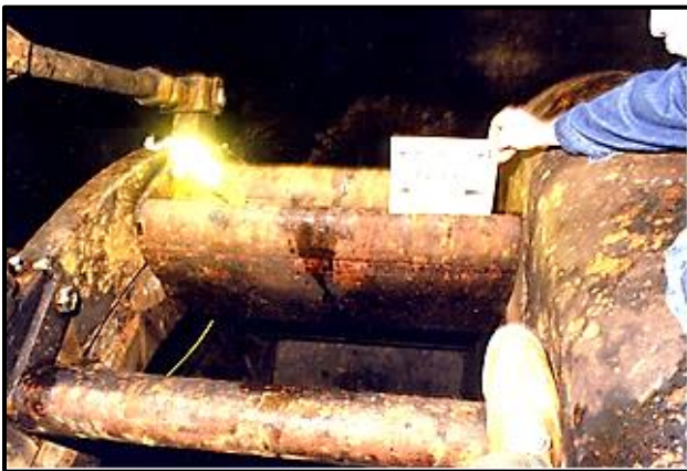
Wicket gates – note, stay vanes inside wicket gates.
