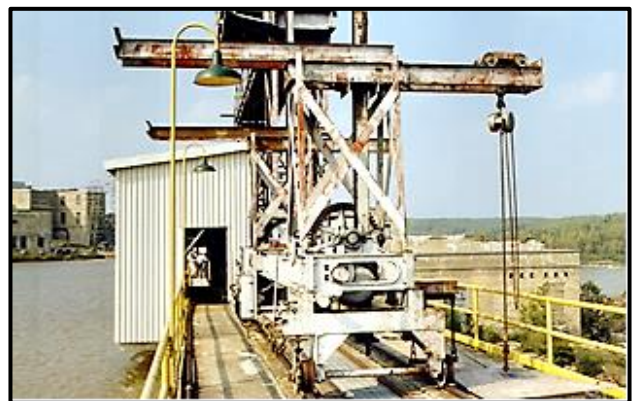
Ancient stoplog hoist – still working.
