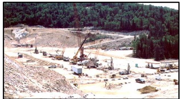
Cut-off wall during construction.
