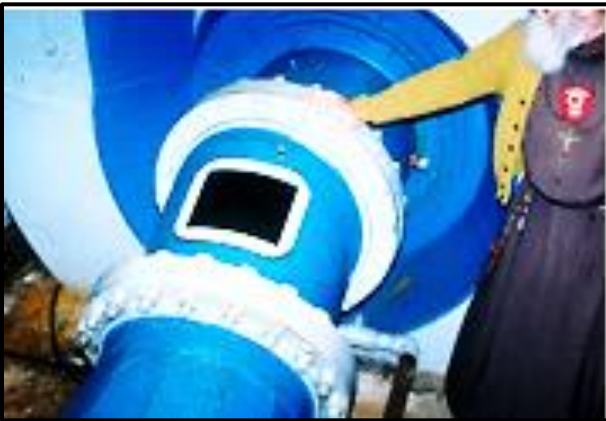
Window in draft tube to observe flow angle.
