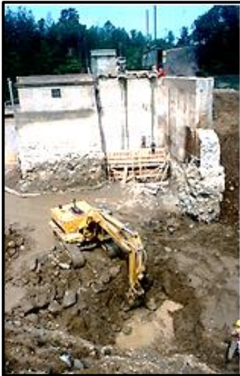
Excavating core trench and placing forms for core contact.
