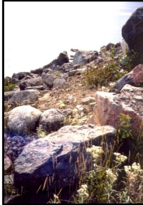
Gap-graded rip-rap on dam.
