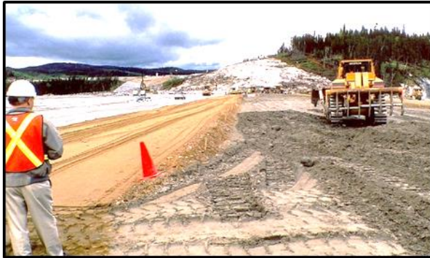
Main dam core placement and upstream filter.
