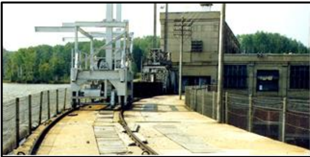
Stoplog hoist. Note spray wall near powerhouse.
