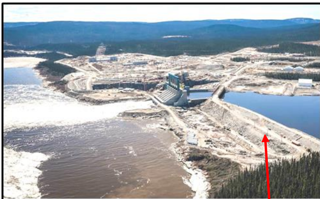
View of Muskrat spillway and cofferdam.
