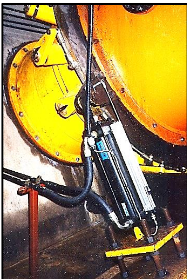
View of turbine servomotor.
