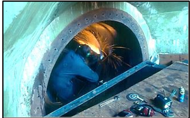
Welding and grinding out cavitated areas.
