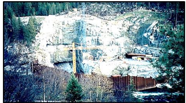
Powerhouse site showing excavation and tunnel adit. Sheet pile cofferdam in foreground.
