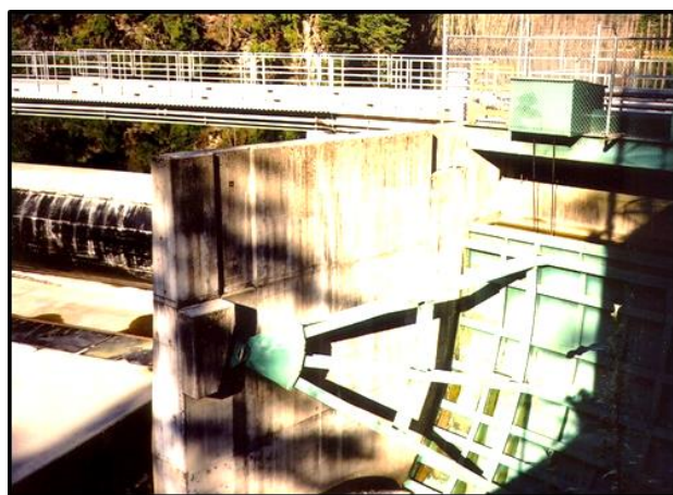
View of Tainter gate low level outlet.
