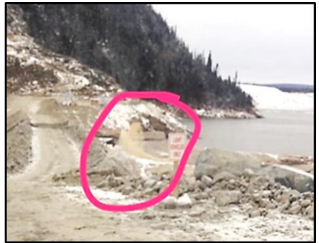
Silty water spout downstream of cofferdam, in center of red circle. Photo by worker on site.
