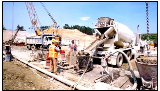
Plastic concrete being poured into cut-off trench.
