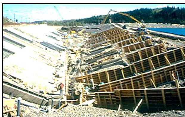
Concreting of weir spillway.
