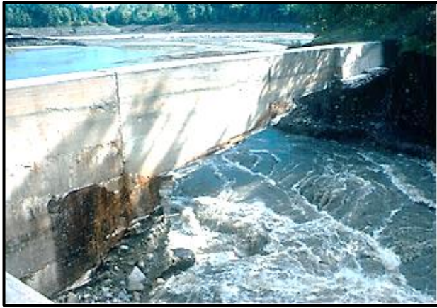
Unreinforced wall over river after washout.
