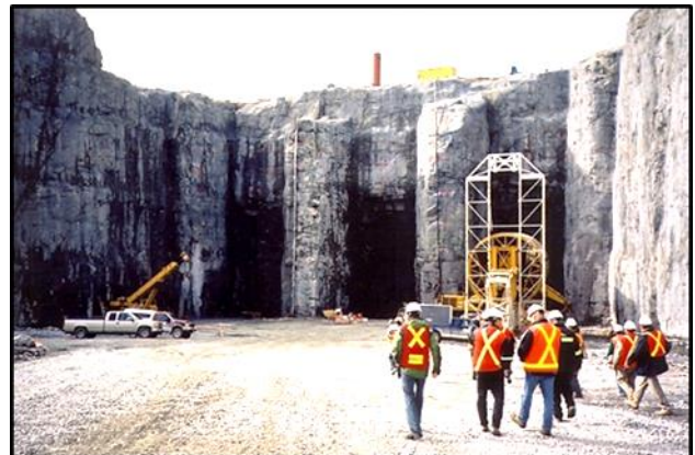
Intake excavation completed, tunnel liner form in right penstock excavation.
