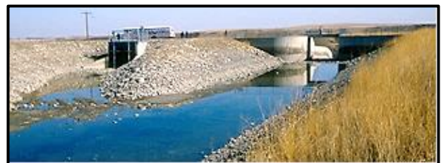
Intake channel, drop structure on right.
