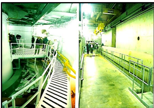
Left – turbine pit. Right – Enclosed draft tube deck
