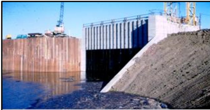
View of intake – headpond half full. Vertical inspection shaft is in square box in corner nearest to camera.
