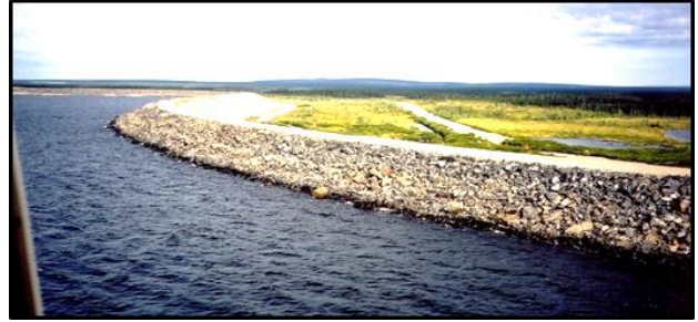
Inspecting rip-rap on Dyke GS-2 at Sail Lake.
