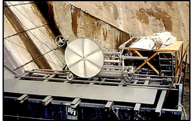
Slot cutting machine.
