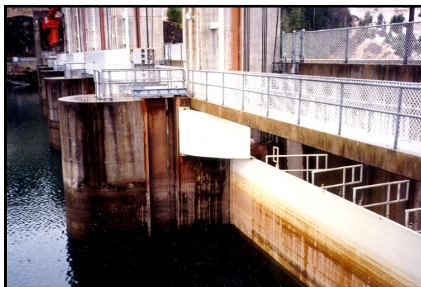
Spillway gate with wave boards on top.
