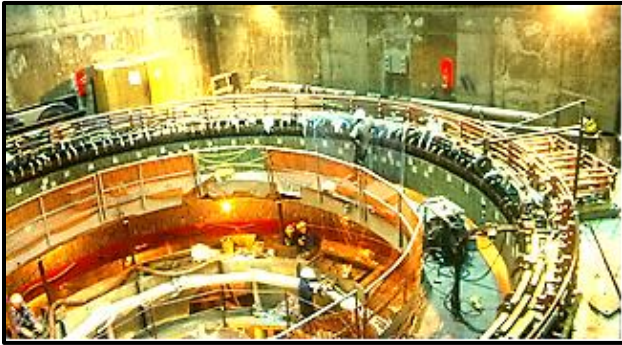
Assembly of generator 12.75m (outer diameter) stator.
