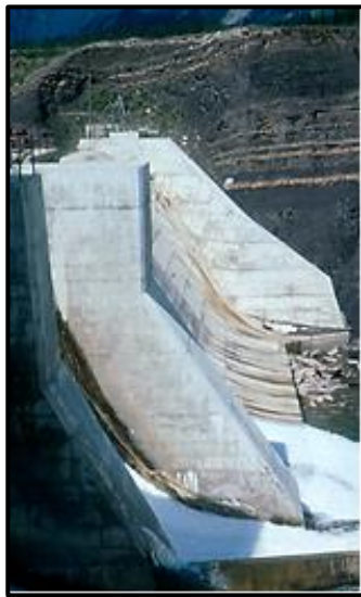
Two views of downstream face, repaired concrete.
