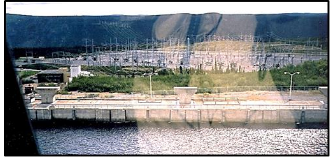
Churchill intakes. Inverted triangular structures are air vents, each one servicing 2 units.
