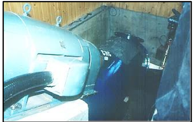
View of generator and turbine. Lever controls wicket gates. Turbines are identical in both plants
