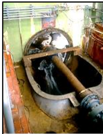
Welding and grinding out cavitated areas.
