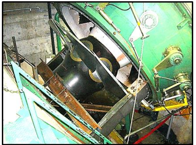
Inclined axis Kaplan turbine.
