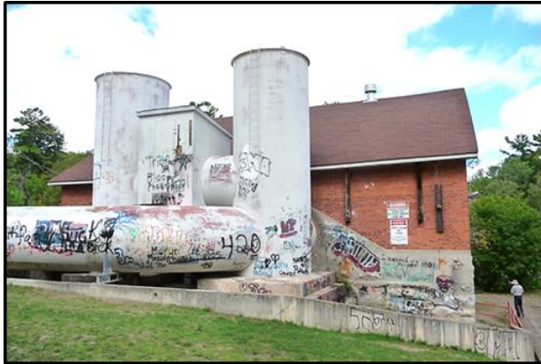
View of second old powerhouse with surge tanks upstream. New powerhouse to be built at side, on grass slope.
