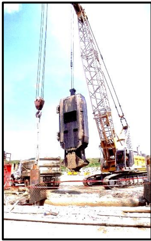
Chisel used to cut through boulders and into rock foundation.
