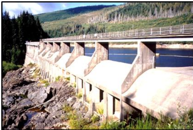
Ambursen Dam spillway structure.
