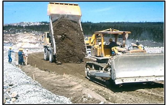
Placing fill near top of dam – a crowded area.
