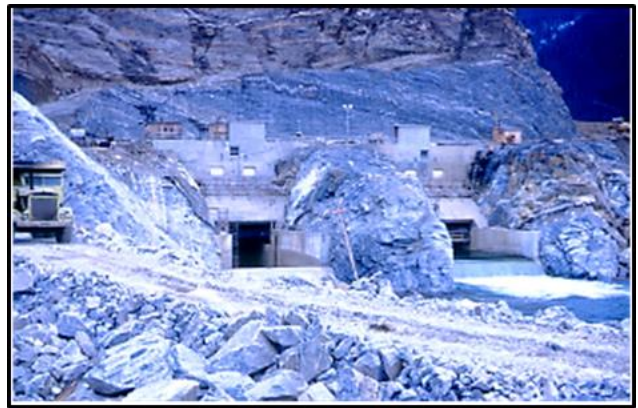
Tunnel outlets with Tainter gates.
