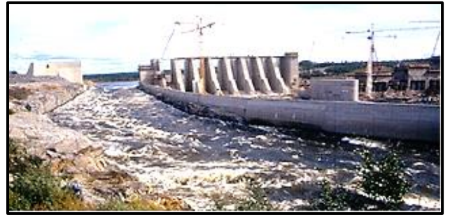
Diversion channel around structures, spillway in center.
