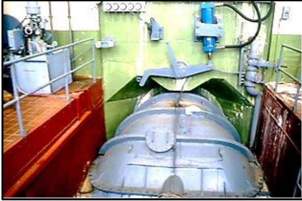
Unit #1. Note wicket gate servomotor above unit.
