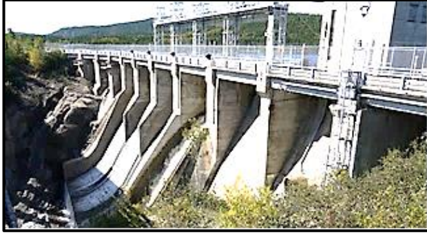
St. Marguerite #2 dam. Source - Panoramio photo. Quick-release stoplogs top left.
