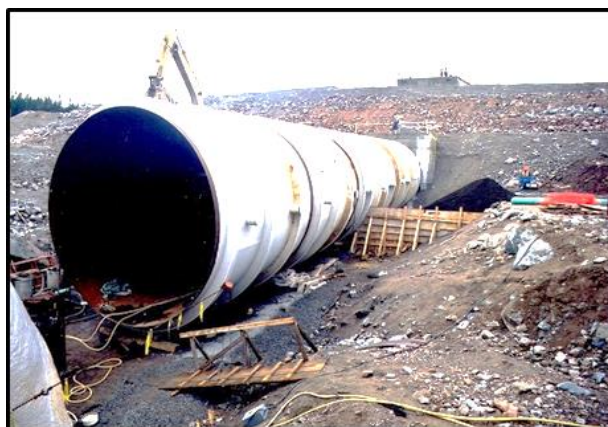
Penstock pipe from intake.
