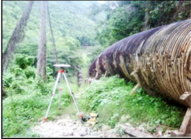
Wood stave pipe - 1998. Photo – Hatch.
