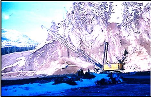
Dragline excavating the slurry trench.
