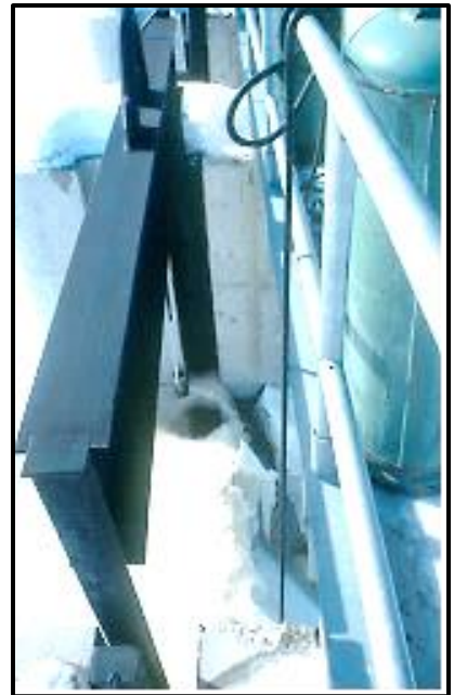
Attempting to melt ice at stoplogs with small propane torch.
