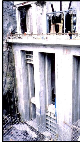
Spillway gate superstructure.
