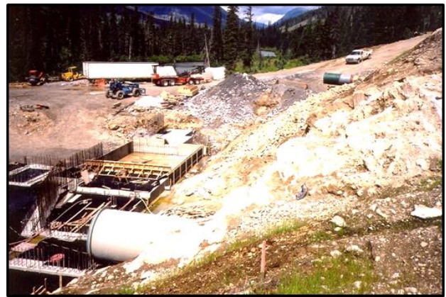
Intake and pipe to low pressure tunnel.
