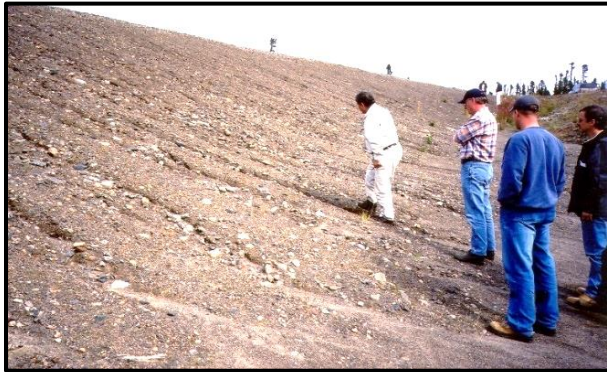
Looking at erosion gullies on GL-27.
