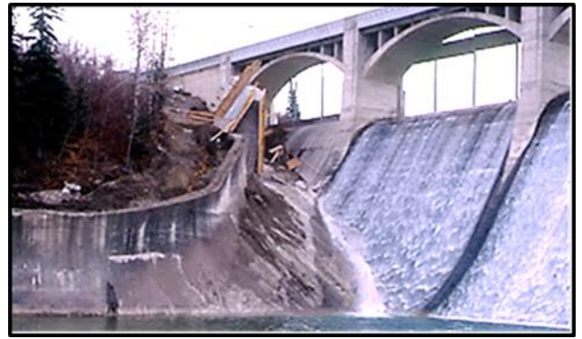
View of right abutment and raising top of training wall.
