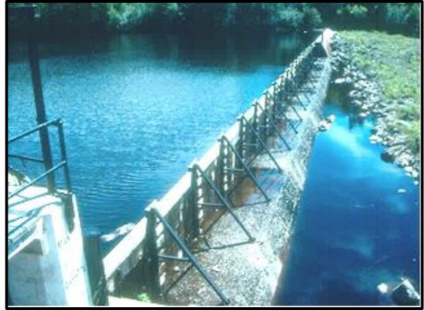
Quick-release stoplog spillway at Weymouth Reservoir.
