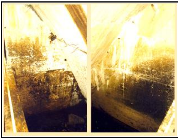
Two views of dam interior, at overflow section. The curved face is the underside of the spillway ogee.
