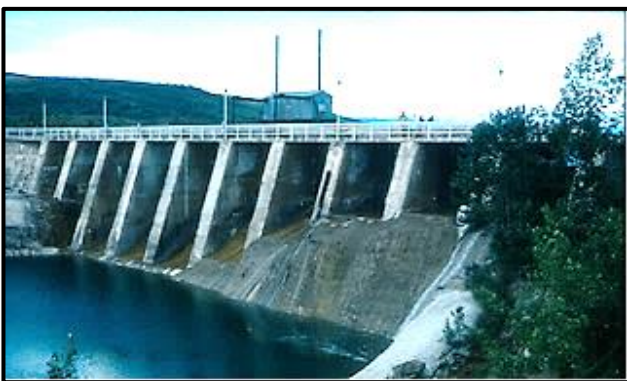
Stoplog auxiliary spillway in side channel.
