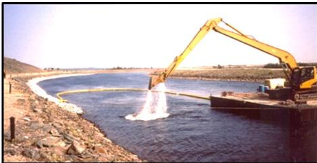
Dumping rock rip-rap to flatten slope. Backhoe equipped with GPS bucket positioning system.
