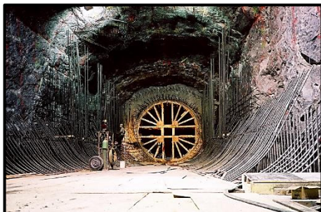
Penstock access tunnel at powerhouse.
