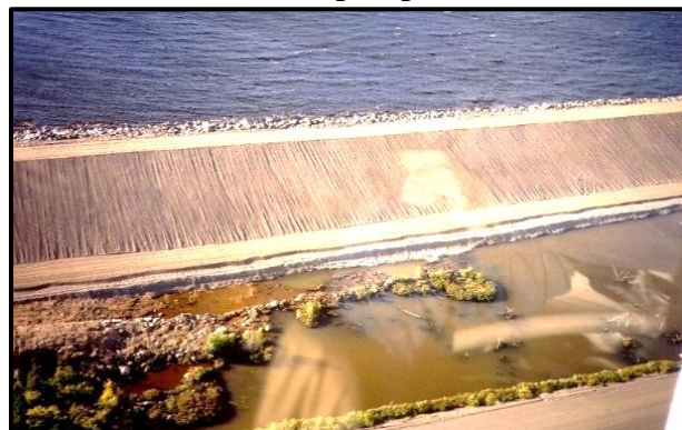
Erosion with even "corduroy runnels" on GL-19.
