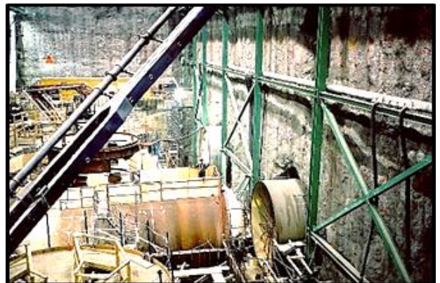
Left - Installing steel spiral casings. Note steel columns from lowest concrete level.
