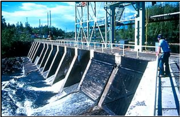
Spillway at Chute Willson. Note flap doors on sluices.
