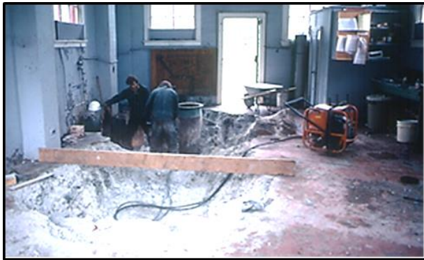
Excavating foundation in powerhouse for larger unit.
