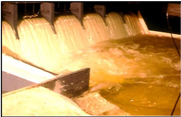
Spillway passing possible maximum flood.
