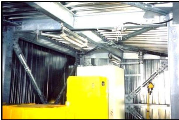
Heavily braced steel housing for hoists.
