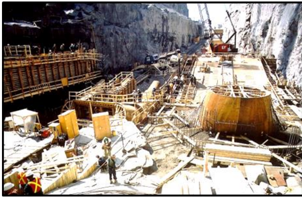
Draft tube form at powerhouse, tailrace rock cut.
