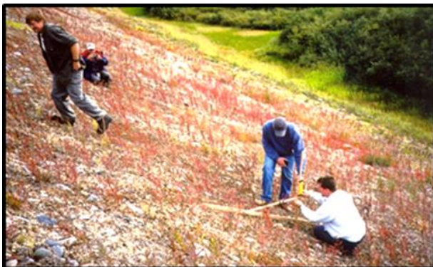
Slope measuring, at 1.8:1 on 5.6km long Dyke GL-31.
