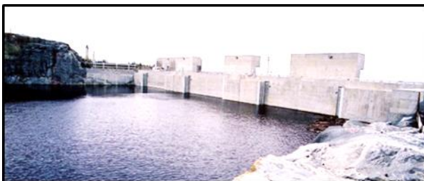
Completed intakes, air vent housing above deck
