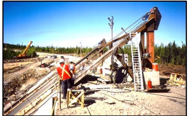
Slip form for the concrete on dam crest.
