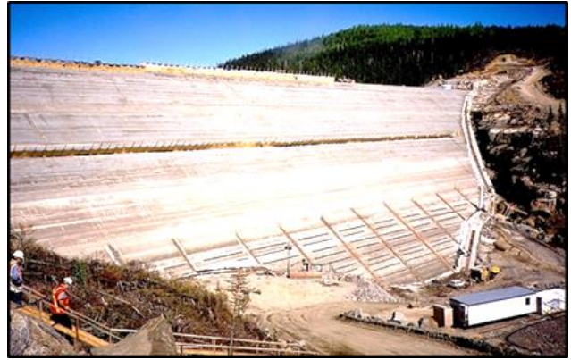
Kerb gaps filled in except near bottom.
