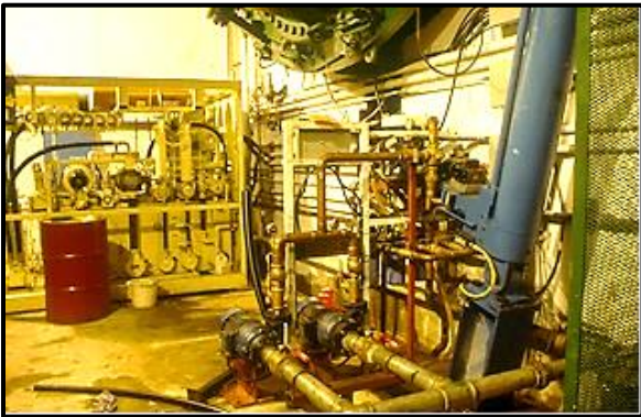
Pumps and piping for operating ring servomotor. Governor at middle left.
