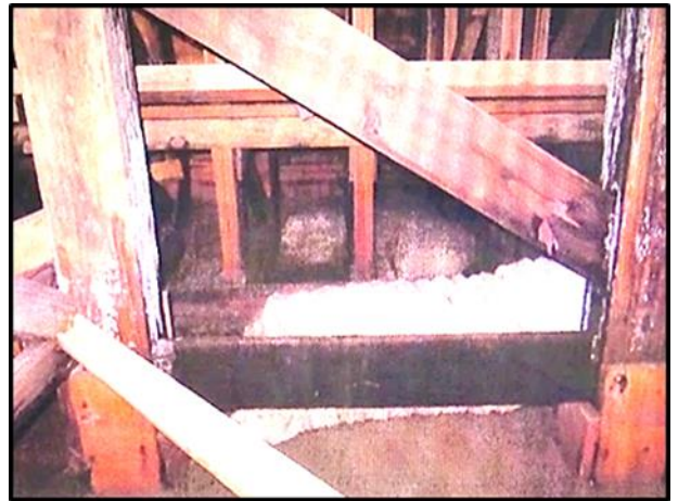
Fungus growth and weathering of timber.
