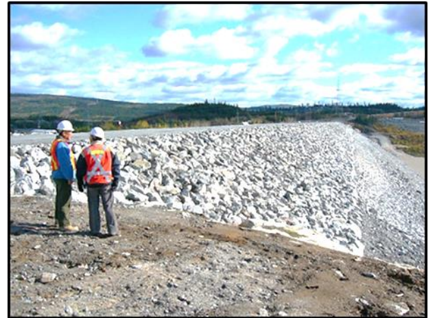
Upstream face of Dyke A. Rip-rap placed with long-arm shovel, not bulldozed, to achieve a smooth face.
