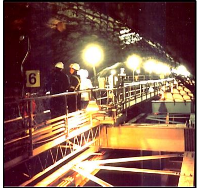
At east end of chamber, overhead I-beam rails for draft tube hoist on bottom right.
