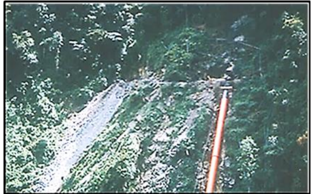
Pipe to side-stream intake at the end of the canal from the Mono Coscapa stream.
