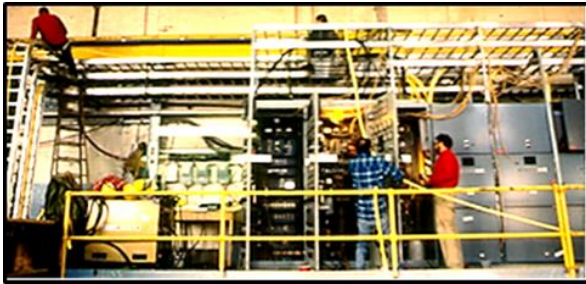
Installing switchgear and controls.
