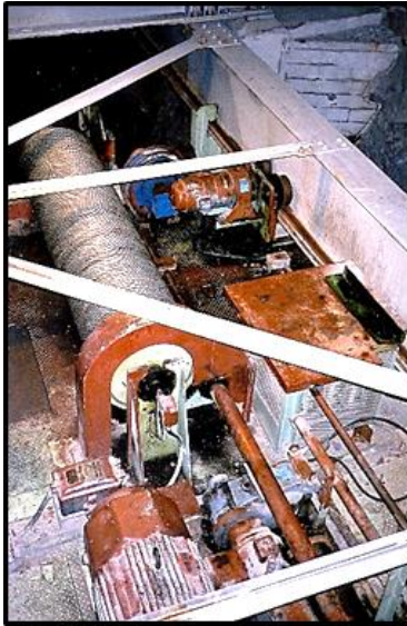
Draft tube gate hoist in surge chamber
