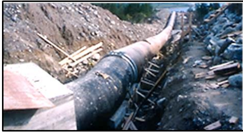
View from intake, short steel pipe to fiberglass pipe.
