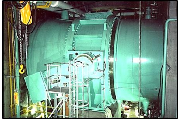
Above - Butterfly turbine inlet valve.
