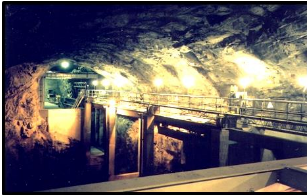
West end of surge chamber showing access chamber.
