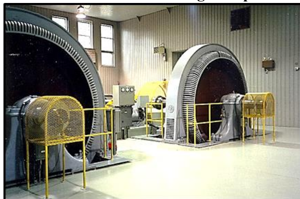
Hydro-Fraser powerhouse with 2-1,062kW units.
