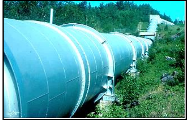
Ring-girder supported steel penstock.
