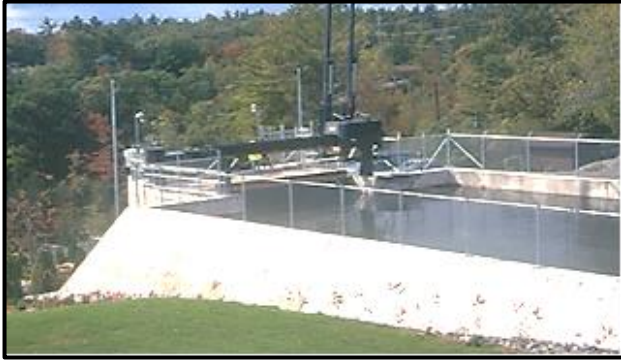
New intake with trash rake.
