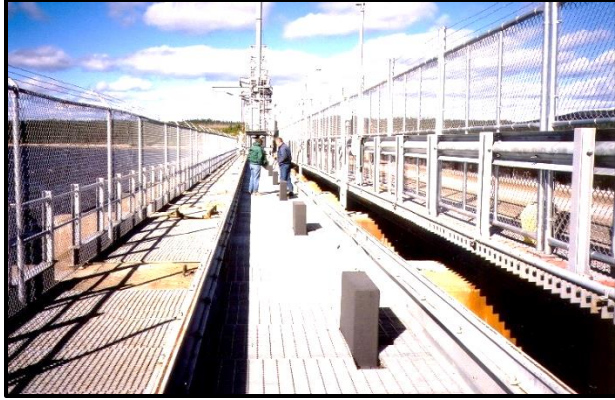
Stoplog hoist deck with locked jacking boxes.
