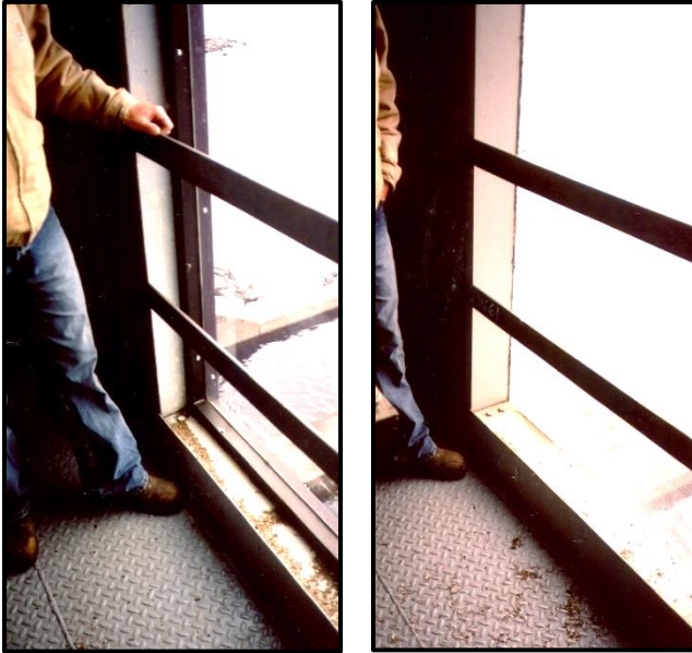
New (right) and old window frame designs.
