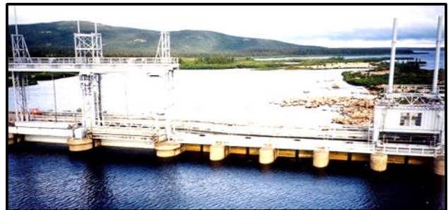
2 screw stem hoist gates on left, stoplog hoist on right.
