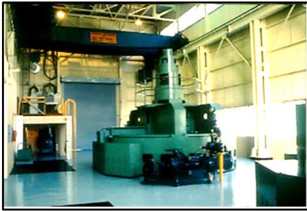
View of vertical axis Francis unit at St. Marguerite.
