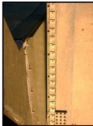
Gate seal jammed against right pier.
