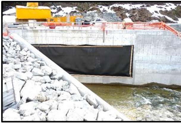
Trashracks with temporary cover to preserve heat inside intake.
