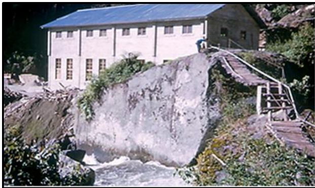
Chururaqui powerhouse set well above flood level.
