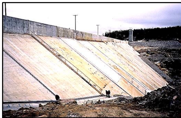
Completed main dam. Note rubber waterstops.
