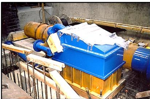
Runner casing for 2-jet impulse unit. Only operates during low flow season.
