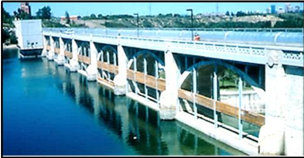
View of dam with new wood gates.
