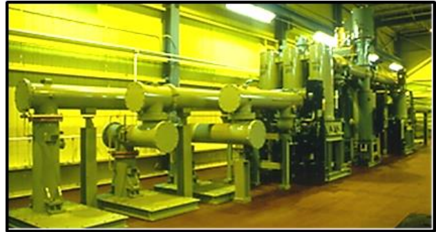
SF6 switchgear – an indoor substation.
