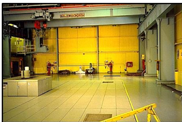
Upper Salmon powerhouse. Generator floor. Note size of generator casing outlined with steel angle painted yellow.
