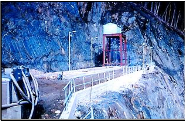
Gantry crane at tunnel intake.
