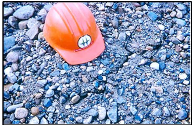
Start of transverse crack across the dam.
