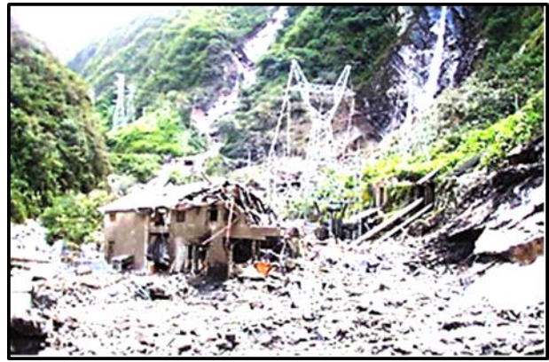
Remains of Santa Rosa powerhouse after landslide.
