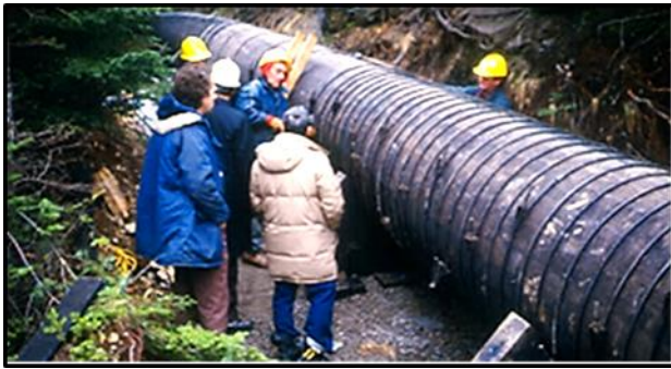
Completing repairs on the wood stave pipe.
