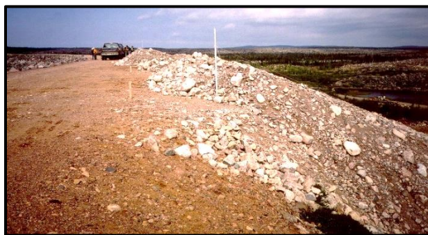
Next year, adding fill to increase height of GR-2 by 1m.
