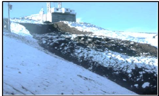
View of earth slide downstream of intake.
