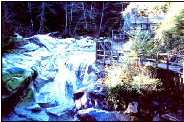
Intake sill and start of wood flume.
